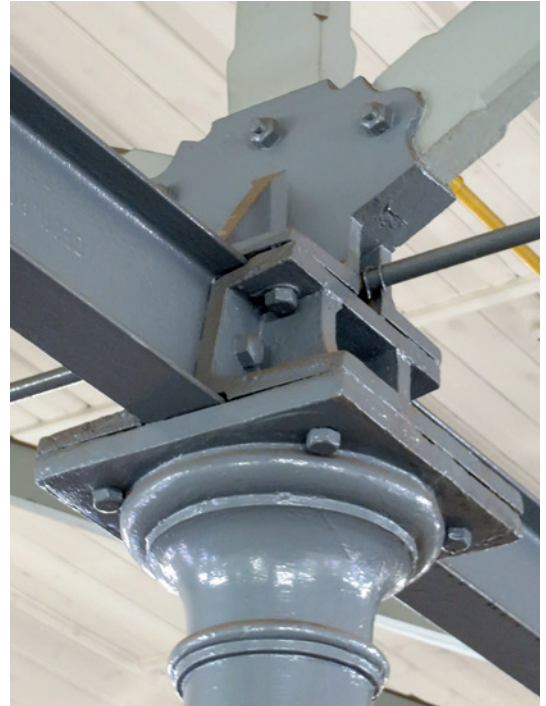
Column capital detail: Precast industrial elements give a special character to the Old Government Printing Works building complex. (Nicholas Clarke)
