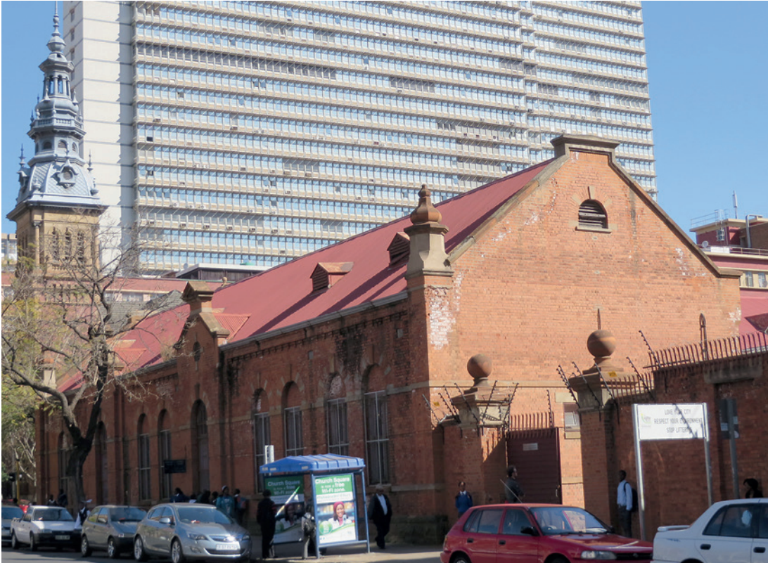
Street view looking up Bosman Street showing the Old Printing Works and the Grootekerk / Melodi Ya Tshwane Church, a unique Eclectic Wilhelmiens ensemble. (Nicholas Clarke)
