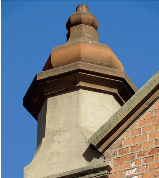
Uninformed restoration leading to accelerated decay. The parapets and gables of the Old Government Printing Works were replaced with a harder brick than the original, leading to further damage. The original face brick gable requires specialist-lead restoration. (Nicholas Clarke)
