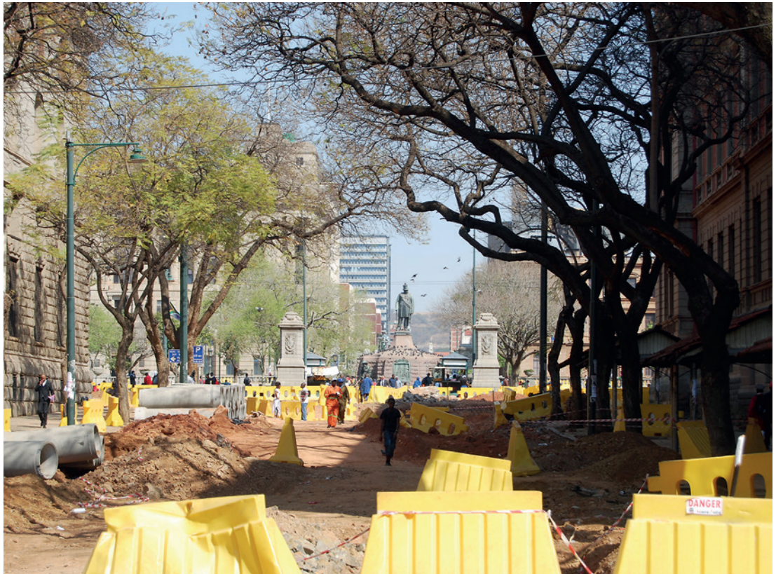
Paul Kruger Street, seen during construction work for the TRT. This will in future become the part of the envisaged Government Boulevard. (Nicholas Clarke)
