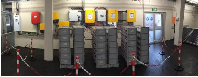
Figure 8 Gen 2 solar-to-hydrogen power converters and 90 kWh battery storage
