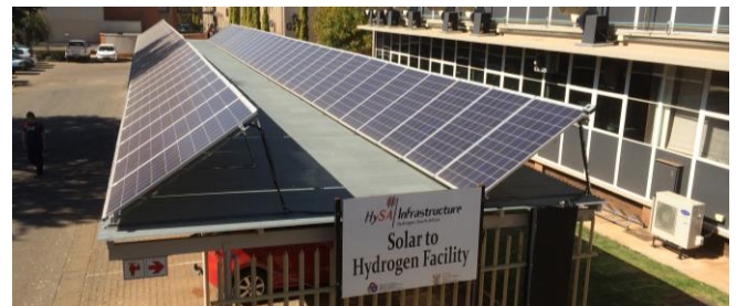
Figure 7 Gen 2 solar-to-hydrogen 15 kW p PV panels
