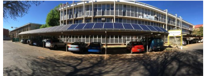
Figure 15 One set of 3kW PV panels cleaned
