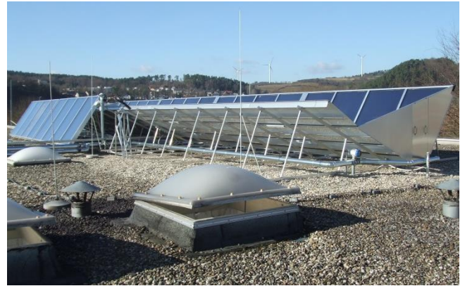
Figure 5: Collector field of the pilot plant at laundry Laguna viewed from east.
