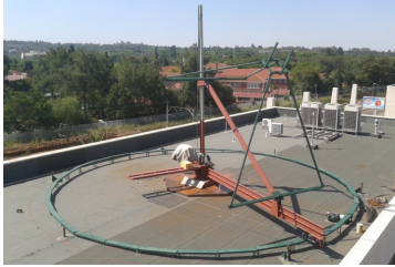
Figure 1 Construction of the two-axis solar tracking system.
