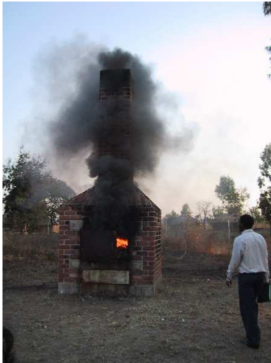
Figure 5: Typical incinerator in operation. Due to maintenance problems, most do not work well.
