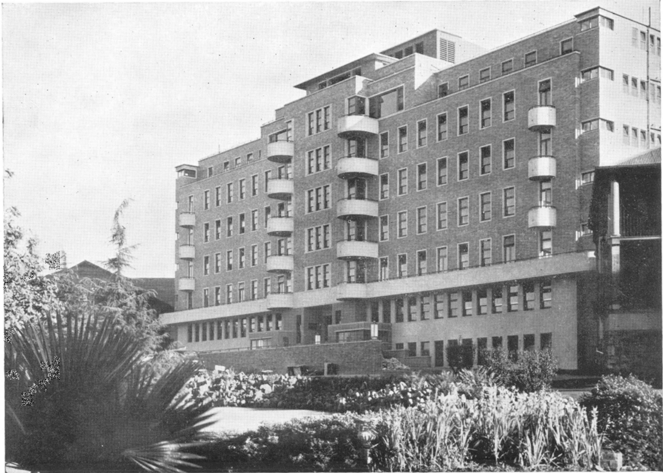
Johannesburg General Hospital (New Block), in which “Selenite” Flush Ceilings were used exclusively throughout. “Selenite” makes the perfect flat ceiling—no joints.
