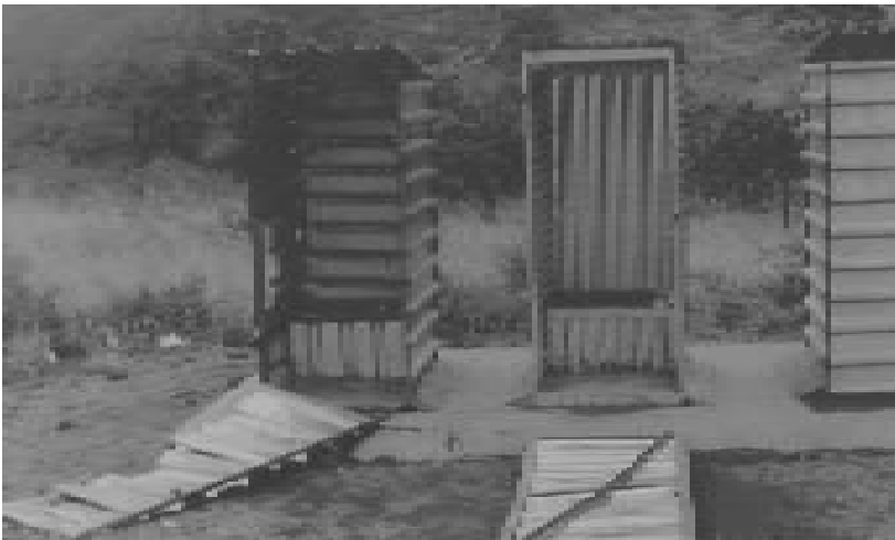
Figure 2 Pit toilets at a rural school
