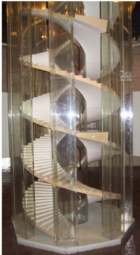
Figure 29 Diagrammatic model of the crossed double stair of the Château de Chambord (source: http://www.leonardo3.net/leonardo/machines_eng.php )
