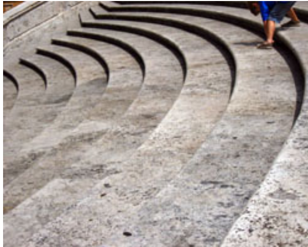
Figure 21 Spanish Steps, detail of steps constructed of cut stone (photograph by the author).
