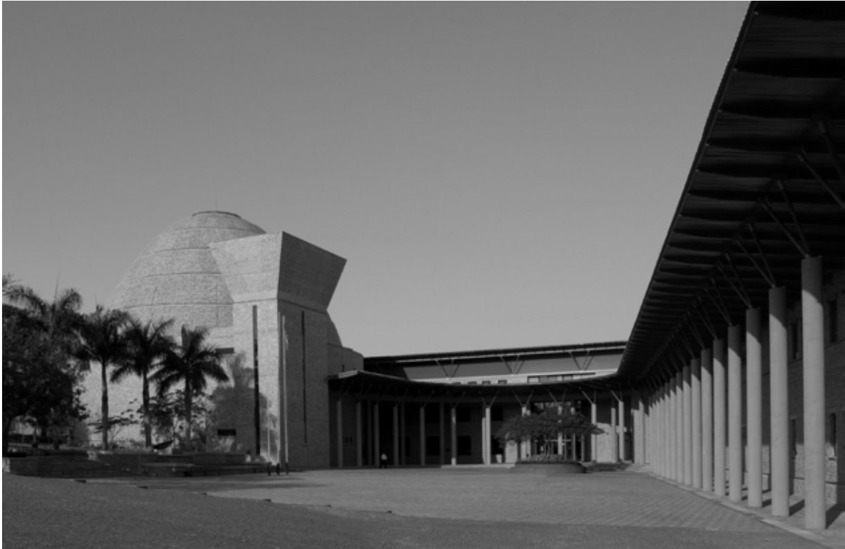
Figure 1 Public square in front of the Assembly, Mpumalanga Legislature in Nelspruit, by Meyer Pienaar, Tayob Schnepel, 1997 (photo: Jonathan Noble 2010).
