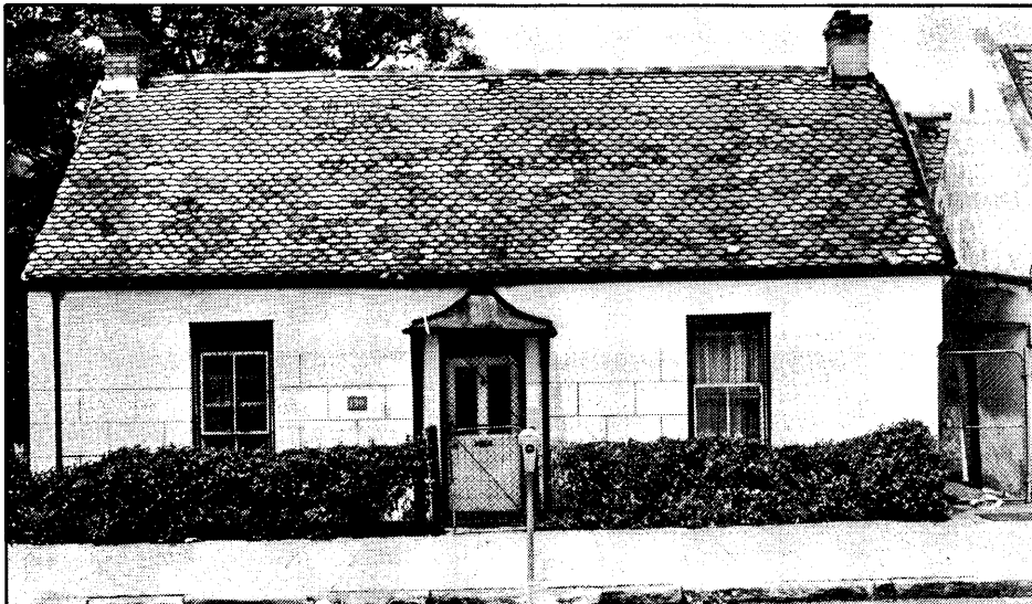
Figure 9: Cottage, 136 Longmarket Street (Moderate Block 15) (1984)
