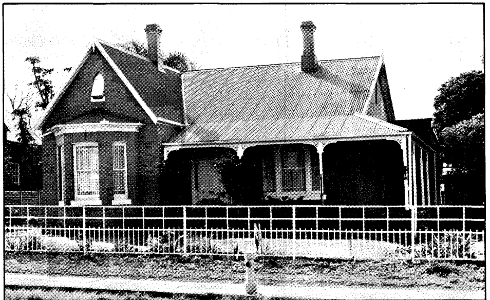
Figure 11: Asymmetrical cottage with bay windows and veranda surrounds, 405 Longmarket Street (Moderate Block 57) (1984)
