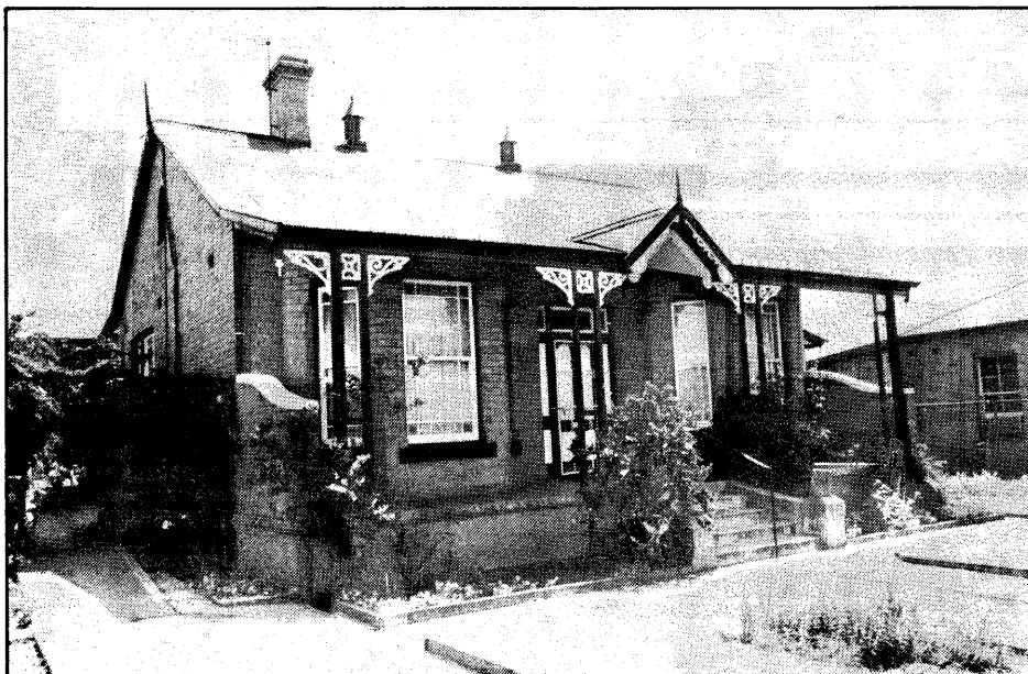
Figure 10: Cottage, 12 Bourke Street, now used for business purposes (Limited Block 54) (1984)
