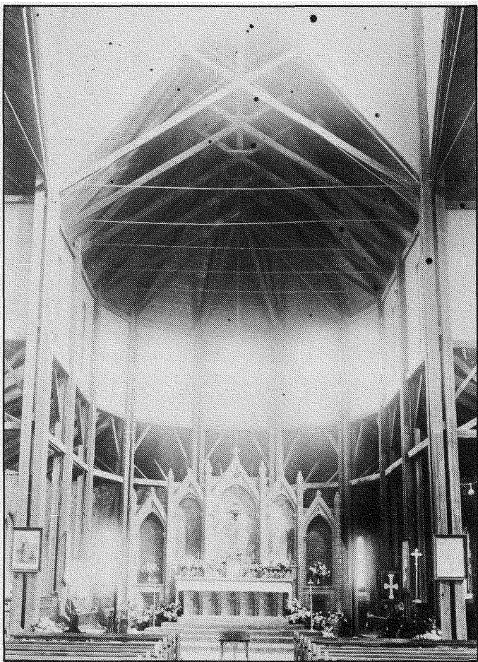
Interior of St Patrick's c 1923. The huge beams of Oregon pine, supporting the roof, are clearly visible.
