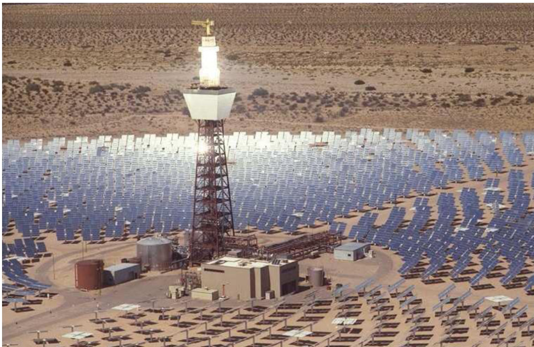
Figure 2-11: An example of a 10 MW CSP in USA (Image courtesy of NREL)
