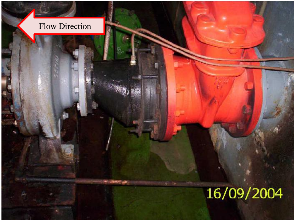
Figure 2.8: Knysna pump station pump inlet piping design together with eccentric reducer (Van der Westhuizen 2011)
