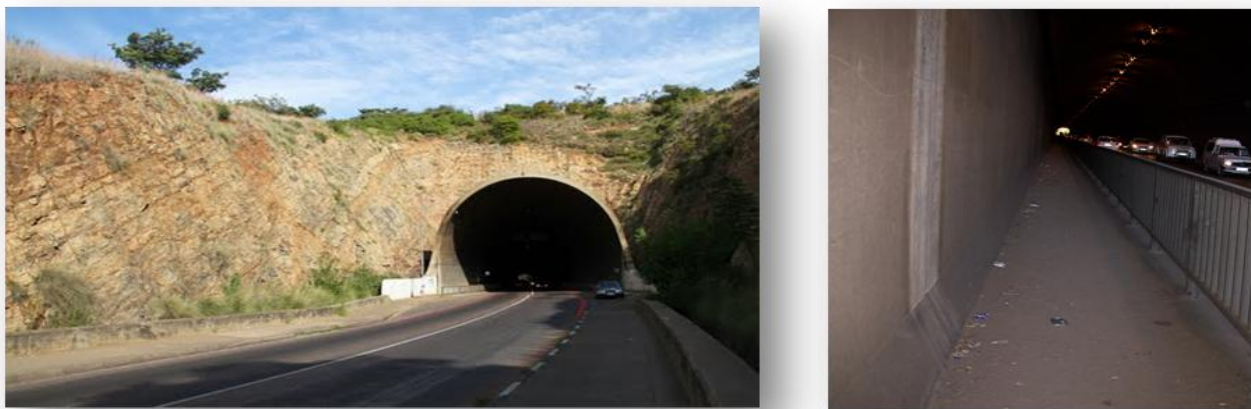
Figure 2-3 Daspoort Tunnel entrance (left) (Photographed by P. Forbes) and pedestrian path inside the tunnel (right) (Photographed by G. Geldenhuys).
