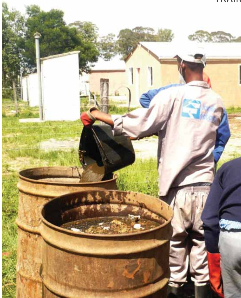
Filling drums with the contents of household pits, after which they are sealed and transported to the safe disposal site
