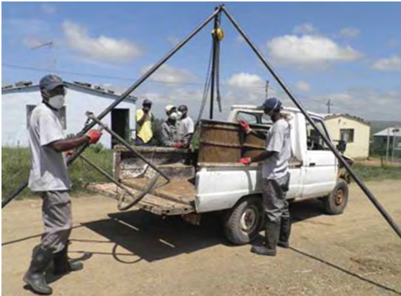
Loading drums, filled with household faecal sludge, prior to their transport to the Dutywa WWTP
