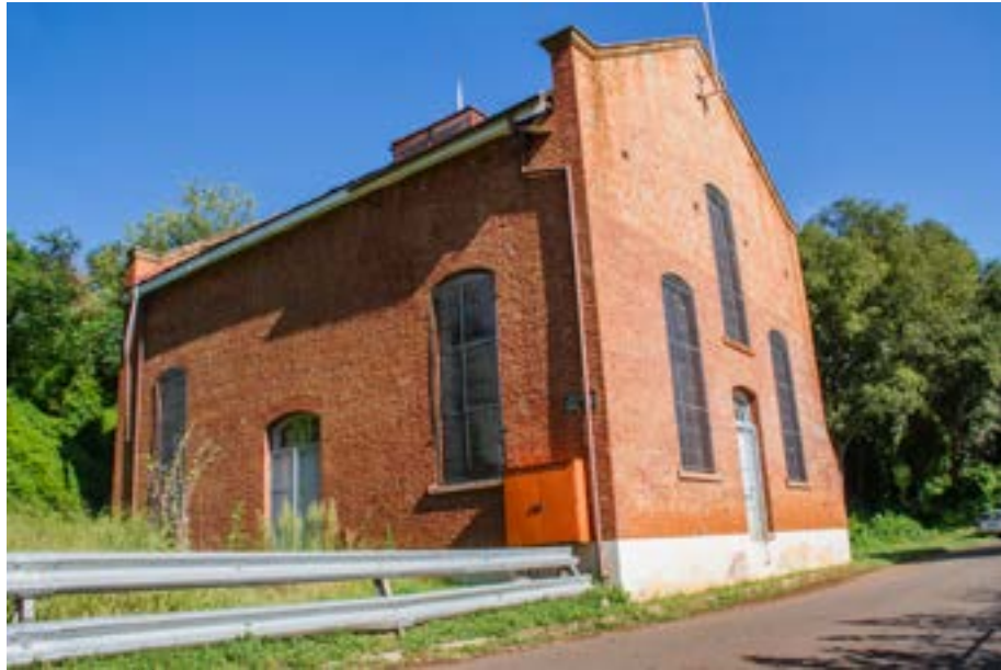
Figure 4.4. (1) Old Pump Station. Photo: Author, 2014.
