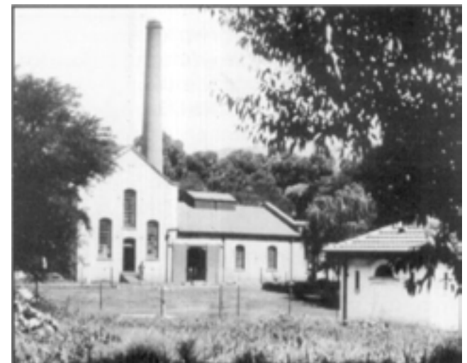
Figure 3.10. Old Pump Station before demolishing of boiler room.
