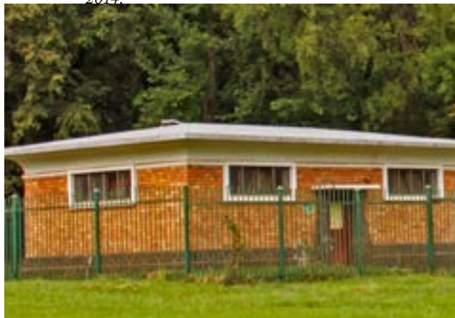
Figure 4.6. (3) Collection & Chlorination Chamber. Photo: Author, 2014.
