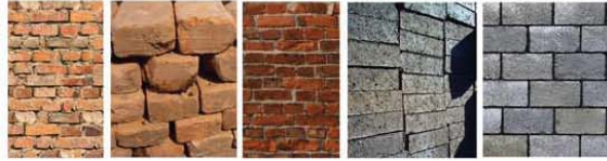
Low quality clay and cement bricks.
