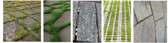
Recycled concrete blocks for pavers, terrace construction and stream stabilisation.
