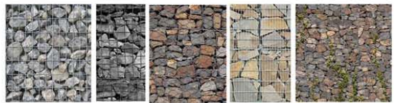
Local natural stone resources used in gabion construction for retaining and soil stabilisation.
