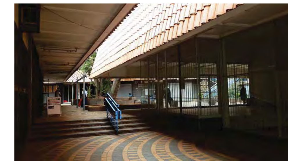
Figure 5.2.5 – Existing stairs at entrance
