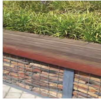
Figure 3.6.4 – Designed benches at Lynnwood Bridge
