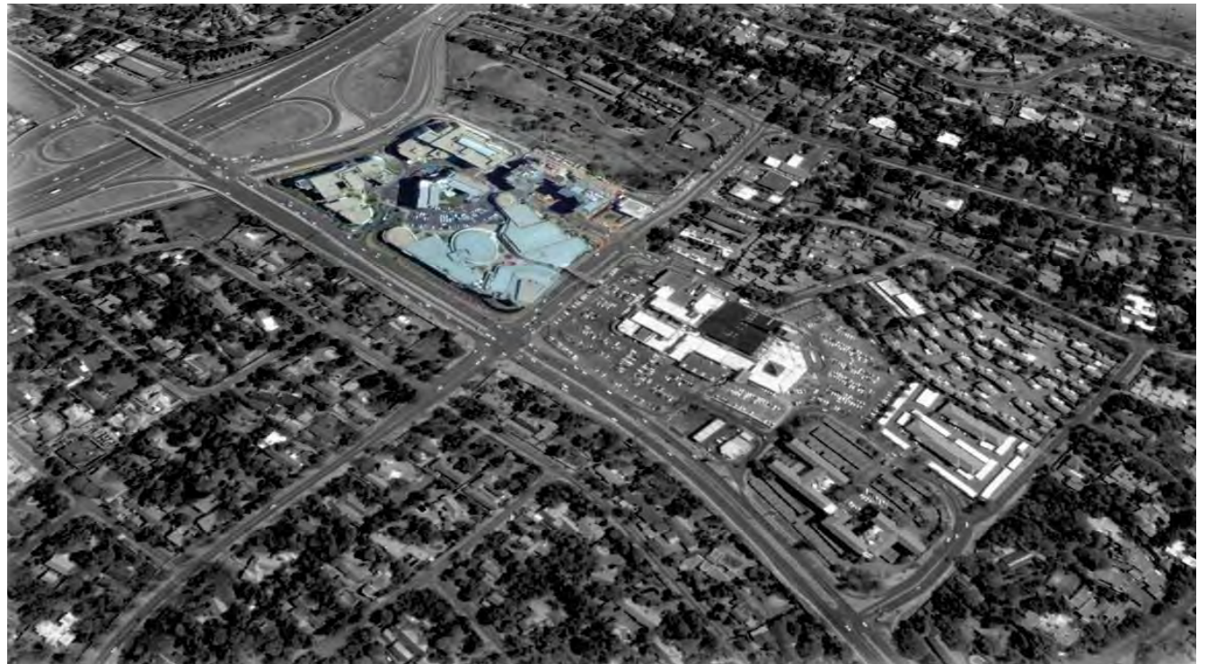
Figure 3.6.3 – Location of Lynnwood Bridge in its immediate context (Google Earth, 2014 with own modifications)
