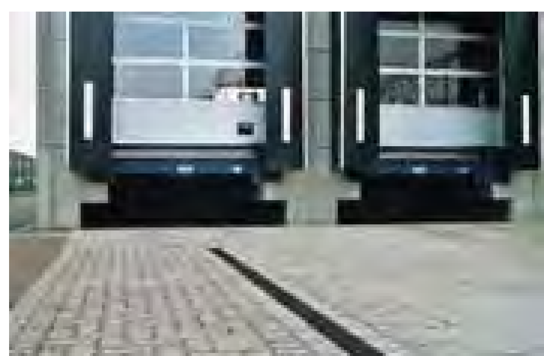
Figure 5.6.13 – Aco Drain Multiline V100-500 with Aco Drain Lightpoint, used as line indicating division between tenant spaces and the courtyard (Aco, 2014).
