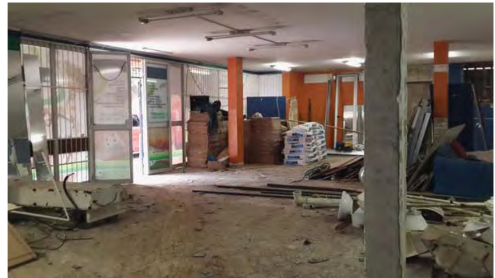
Figure 4.4.32 – View of Block A's interior (mystery space)
