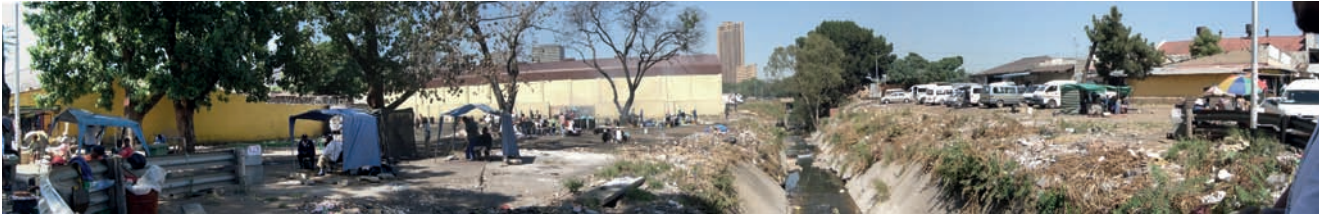
FIGURE 6 The canalised Steenhovenspruit and surrounds, in 2013 (Cronje, 2013: 69).
