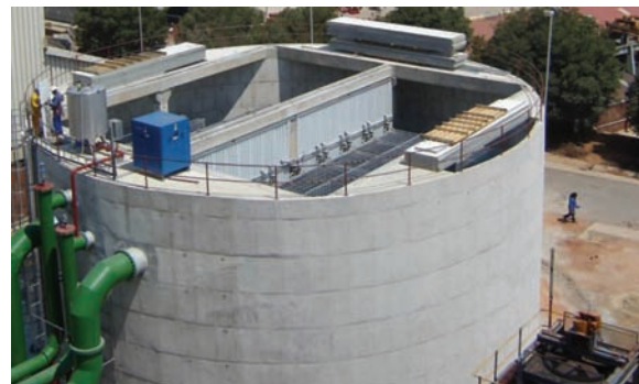
Figure 2— Ice storage dam
