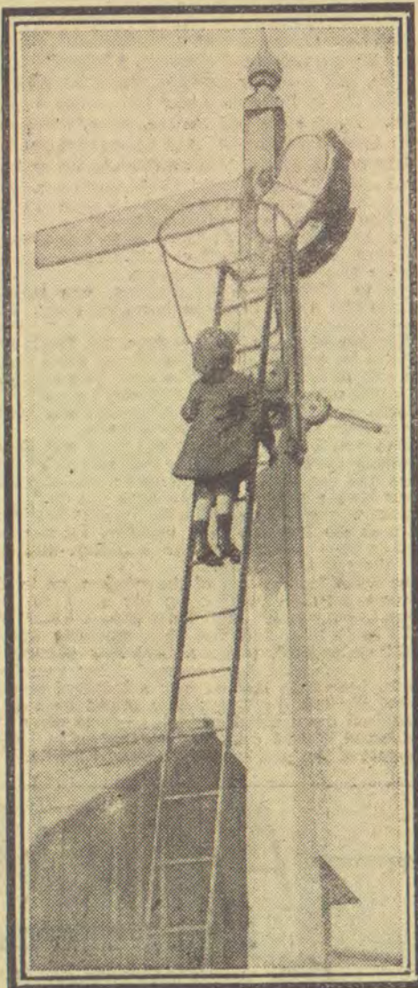
Seeing the signal lamps are lighted.
