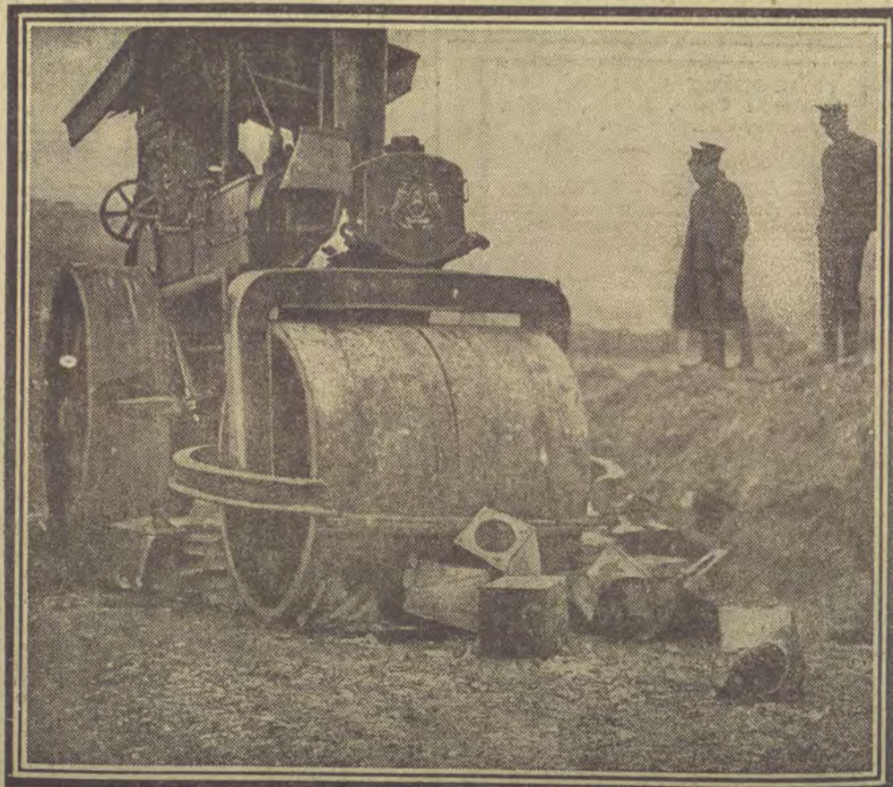
To provide material for munitions tin cans are now being crushed under steam-rollers. Every little helps to the crushing defeat which awaits the Hun.
