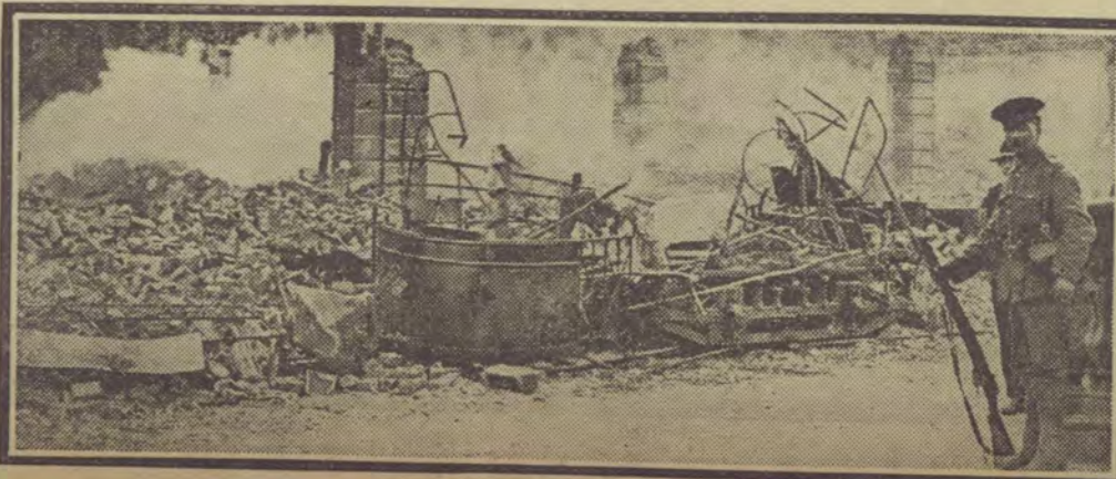
A city tramcar, used as a barricade, was destroyed by the fire.
