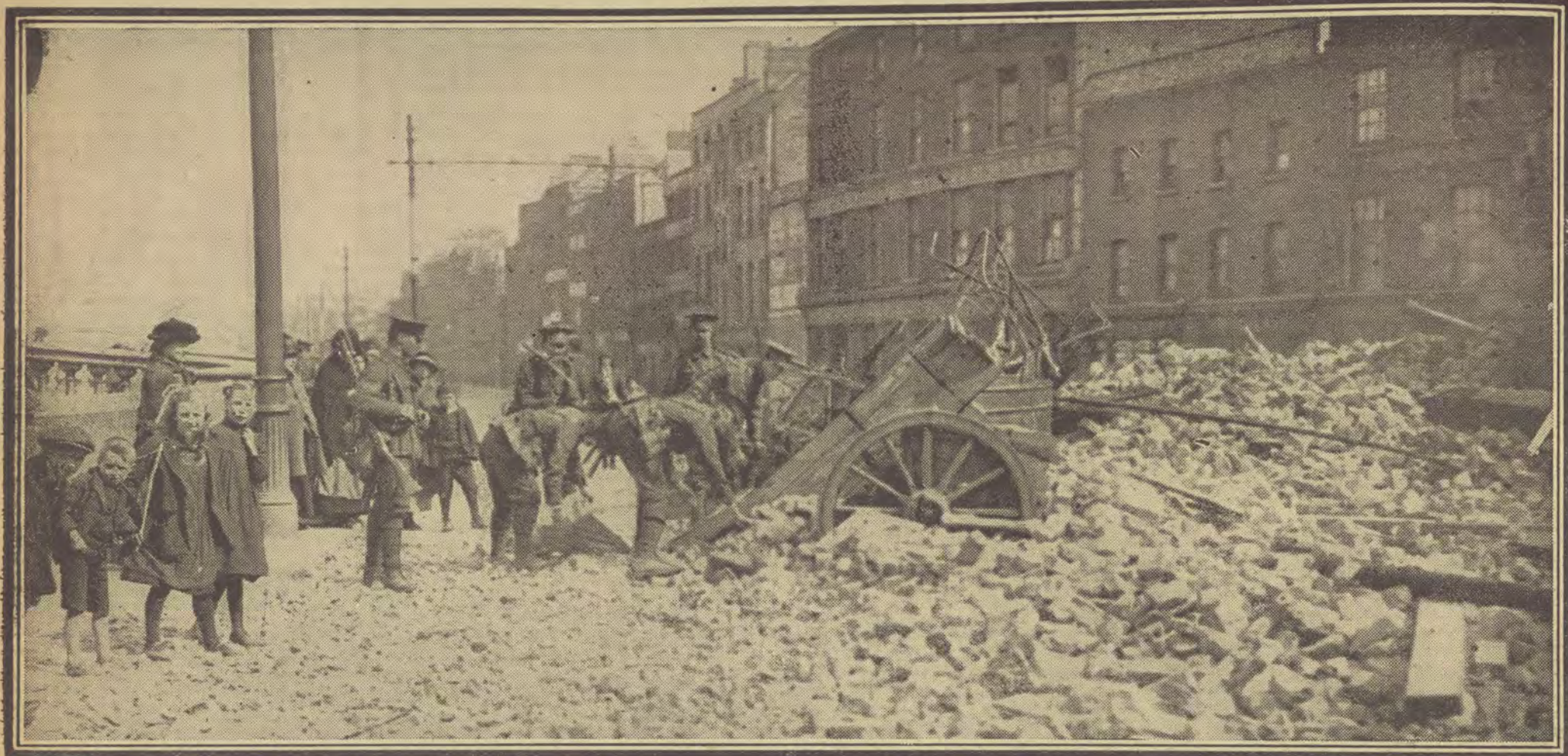
Soldiers clearing away the debris that blocked Church-street Bridge. Some of the streets were absolutely impassable on account of the fallen masonry.—(Daily Sketch Photo.)
