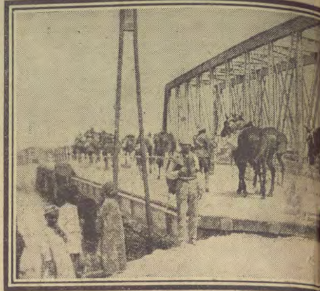
Troopers of the Dorset Yeomanry, who distinguished themselves at their quarters at the base. The railway bridge which they crossed is their first contact with civilisation after many months.
