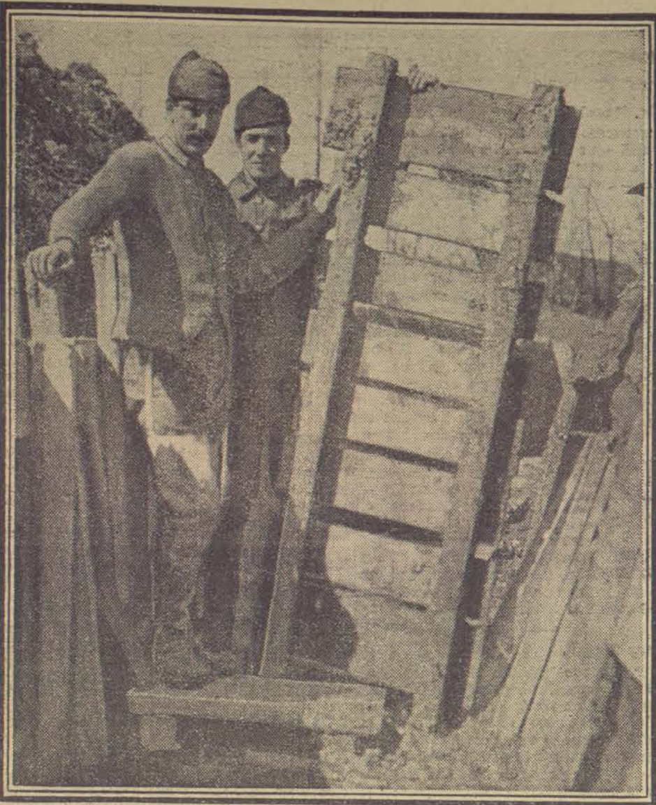
When Tommy finds it necessary to bail the water out of his flooded trench he raises the wooden flooring which helps to keep his feet dry.
