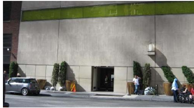
Figure 4.17 Hudson Hotel, Facade (Hudson Hotel, 2012)
