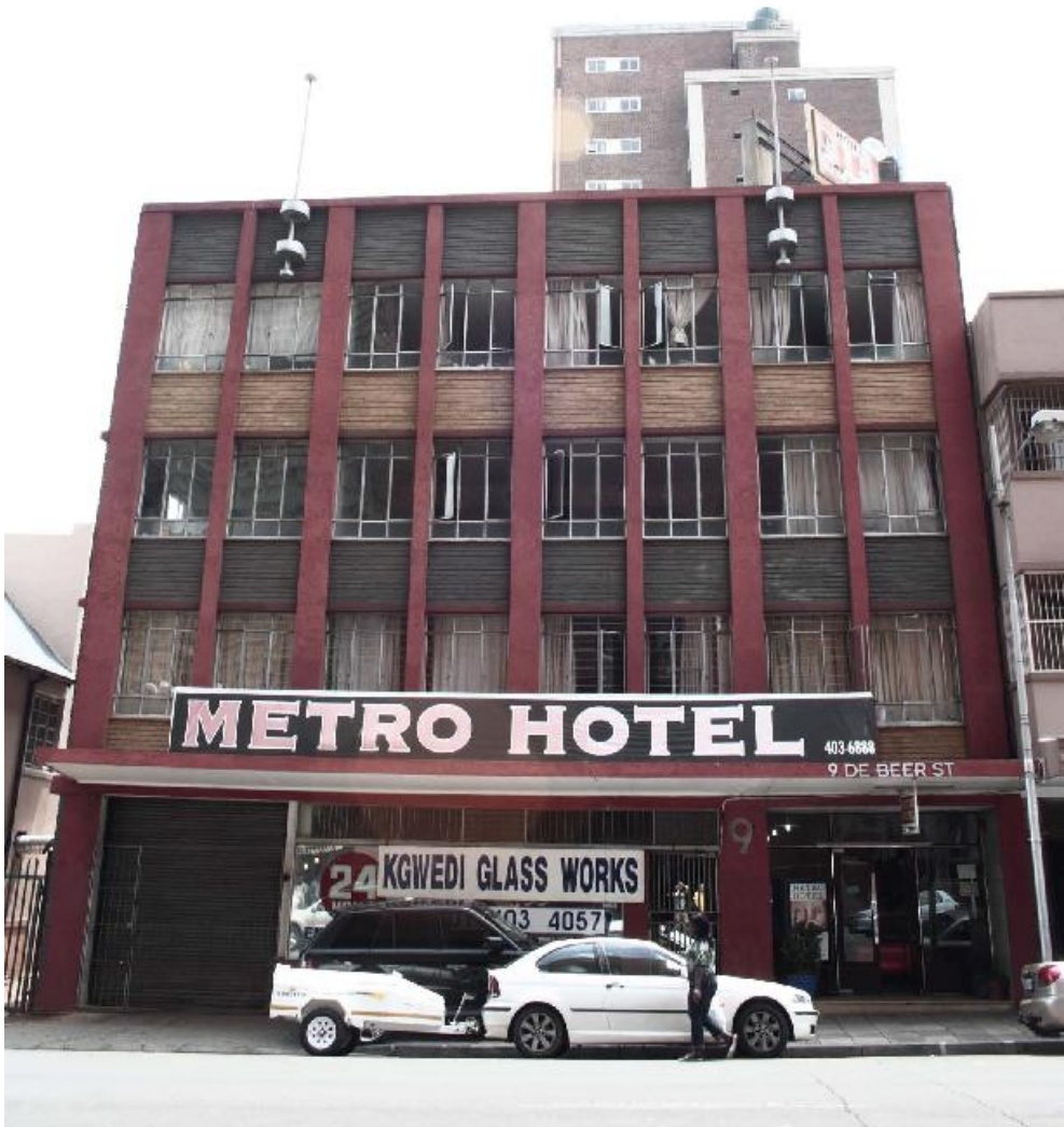
Figure 2.36 Eastern elevation of building (Strydom, 2012)
