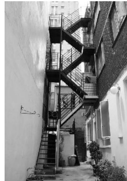
Figure 2.38 Courtyard on western end of building (Strydom, 2012)
