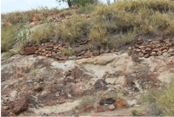
Fig. 4 Retaining walls of the “palace” on top of Mapungubwe Hill (photo: S. Chirikure)
