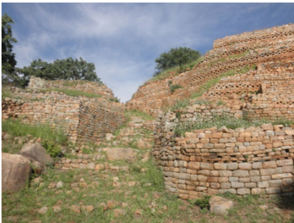
Fig. 5 Retaining walls on the Hill complex at Khami. Note the multiple bands of check decoration (photo: W. Ndoro)
