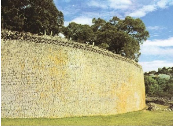
Fig. 6 Example of freestanding walls at Great Zimbabwe, the outer curtain wall of the Great Enclosure. Note the chevron pattern at top (photo: I. Pikirayi)
