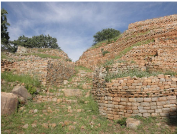
Fig. 5 Retaining walls on the Hill complex at Khami. Note the multiple bands of check decoration (photo: W. Ndoro)
