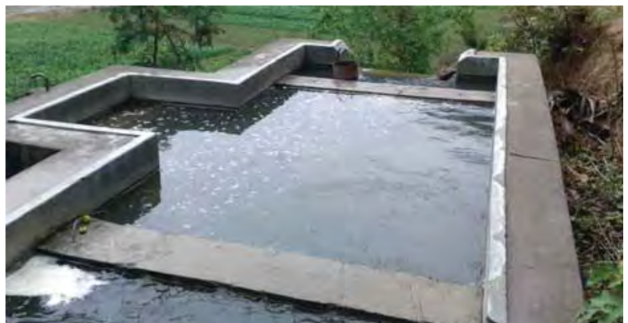
Figure 3: Intake collecting water from stream
