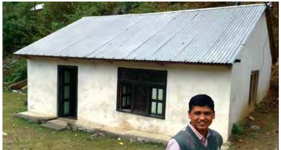
Figure 2: Turbine room, Karamdanda project, Nepal
