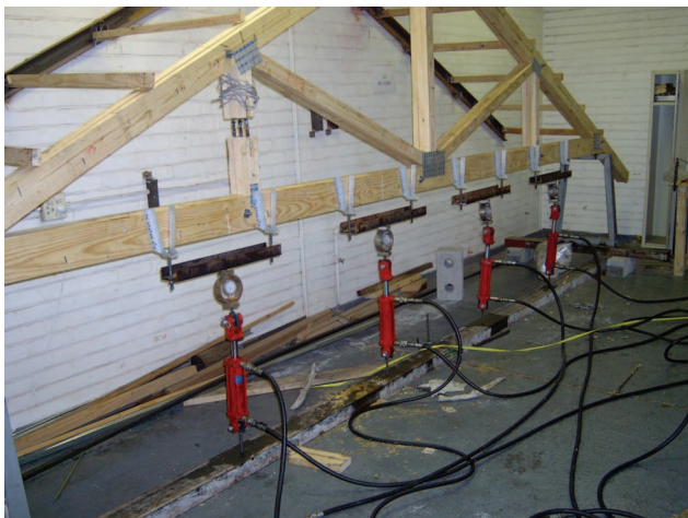
Figure 9. The relative positioning of the loading jacks and the flexible load cells
