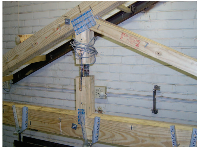
Figure 7. This shows the specially prepared calibrated load cell placed in the web members
