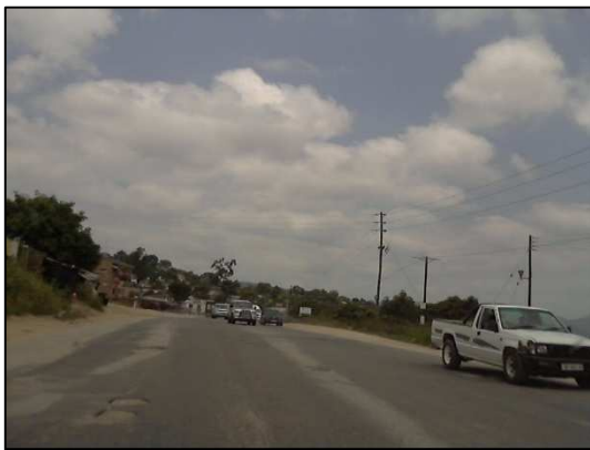
Figure 5-4: Surface Failures km 27.84 R538(2), SRT (2013)
