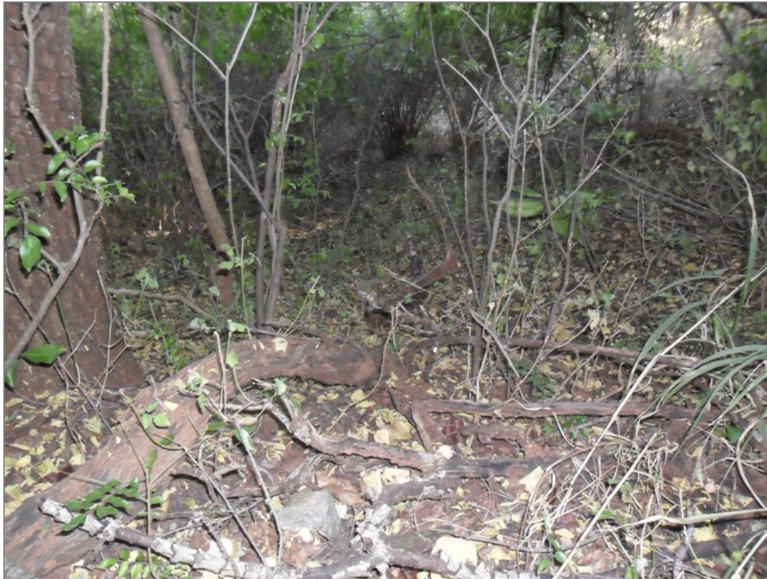
FIGURE 29: Photograph taken of the drainage channel at point 11 showing bare roots from larger plants.
