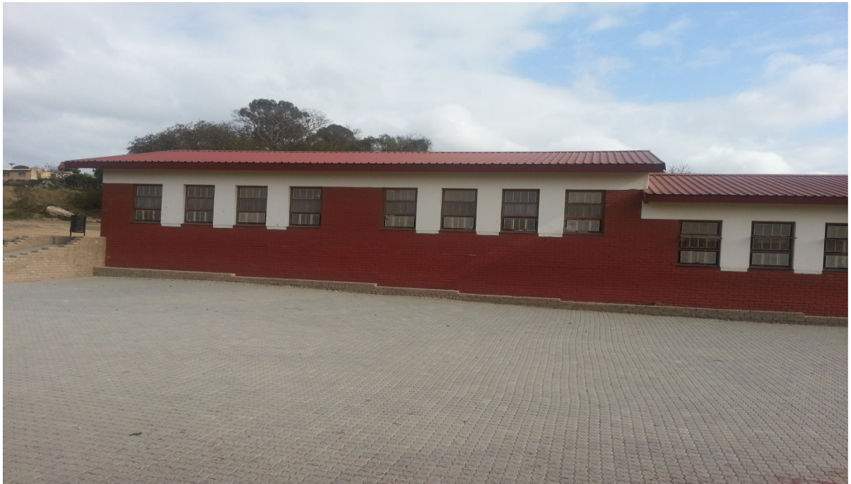
CLASSROOM BLOCK IN SCHOOL B
