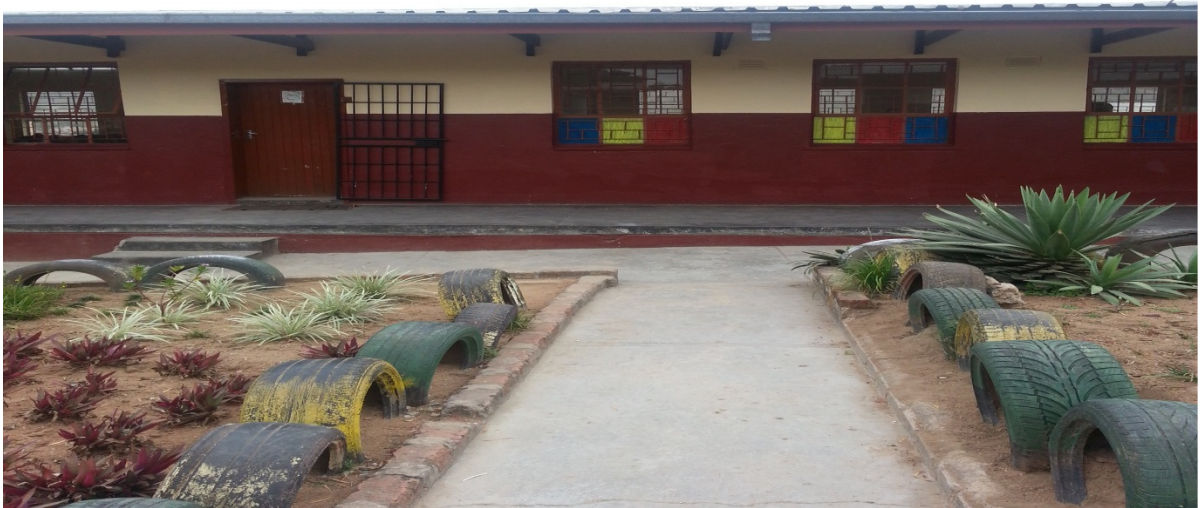
CLASSROOM BLOCK IN SCHOOL D
