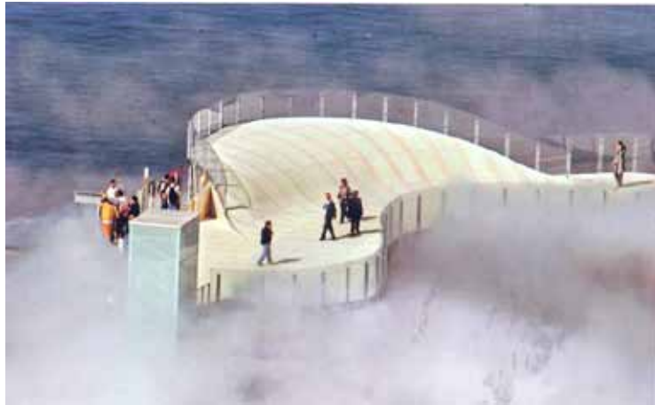
Figure 12 Diller + Scofidio, Blur Building , Yverdon-les-Bains, Lake Neuchatel, Swiss Expo 2002 (source: Aymonino 2006).
