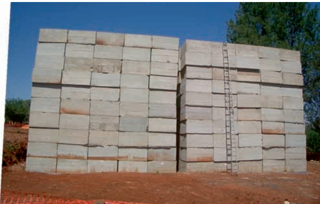
Fig. 4. The first surcharge stack shortly after completion.
