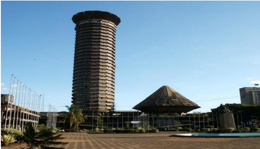
Fig.4b: Karl Henrik Nostvik. Kenyatta International Conference Centre, Nairobi. 1973. A view of the KICC ground plaza in the foreground. The key elements of the architectural composition are also evident. The podium, the cylindrical tower and the conical amphitheatre are perceived in harmonious unity. The alternating horizontal bands on the main tower as well as the helipad atop the tower can be identified with clarity. (Source: kenarchworldpress.com).
