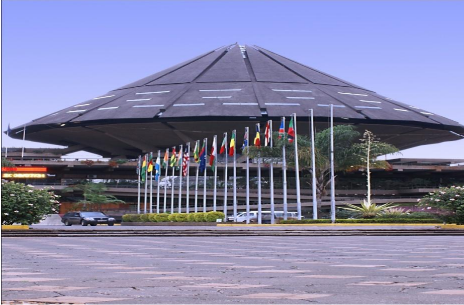
Fig. 4h: Karl Henrik Nostvik. The Amphitheatre at KICC, Nairobi. 1973. Note the conical pyramidal roof with roof lighting effect (Phenomenology: dimensions of natural understanding). The ramps on the podium level are evident as well as the multiple flags of various nations indicating vibrancy of experience through circulation and multiple temporary identities.
