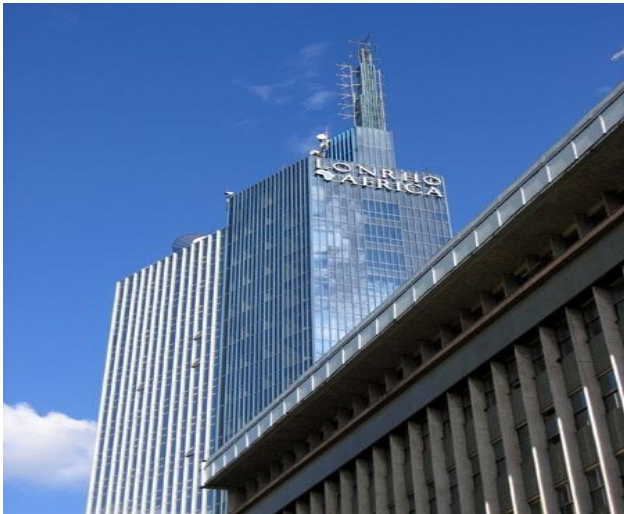
Fig.21v: Planning Systems architects. The Lonrho House, Nairobi. 1990. The architects James Archer and Trevor Andrews designed the building facing significant site constraints. The extensive use of glass can lead to a 'green house' within the tropics requiring inappropriate use of artificial air conditioning.
