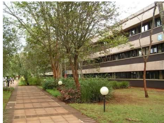
Fig. 2u. Mutiso Menezes International. The United Nations, Gigiri. s.a. A harmonious composition of low key buildings in a humanized configuration.
