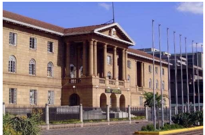
Fig. 21o: Herbert Baker. The High Court, now The Supreme Court, Nairobi. 1934. An exemplification of neo-classical architecture, a harmony of the Doric Order, arches, stone masonry in grandeur.
