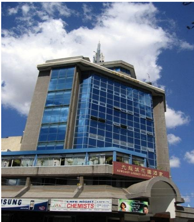
Fig 23h: F. G. Mungai, AAKI architects. The Ngingo Towers, Koinange street, Nairobi. 1995. The artefact relates positively to the street.
