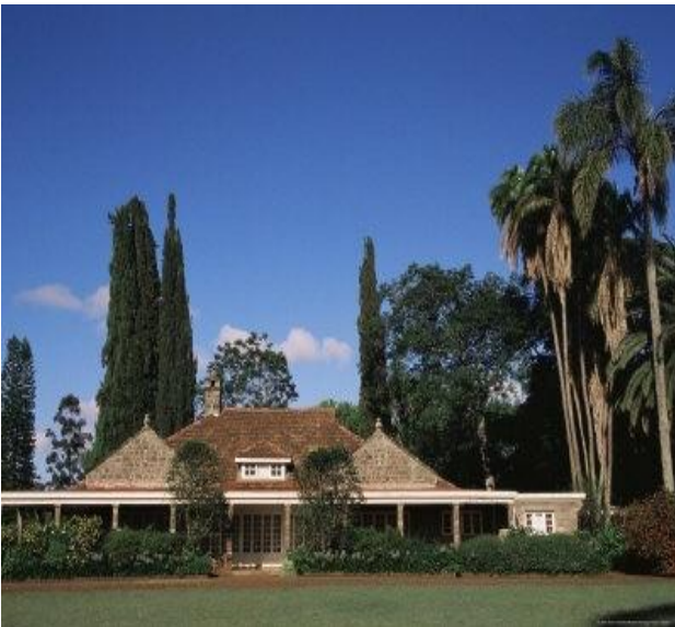
Fig. 21r: Ake Sjorcken, arch. The Karen Blixen residence, Karen, Nairobi. 1928. The artefact is now part of the National Museums of Kenya. The long colonial verandah is evident, as well as the English dormer window. The hipped and gabled roof creates further visual harmony of form.
