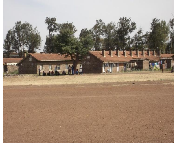
Fig. 21q. Chief architect, Kenya Railways. Makongeni Estate, Nairobi. s.a. Detached units in a linear configuration. Each unit contains several houses within it. This estate portrays the colonial mindset regarding the lack of individuality by the Kenyan native, justified by the colonial prohibition of workers' families in urban areas.
