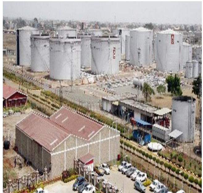
Fig. 2m: Architect unknown. Kenya Pipeline, Industrial Area, Nairobi. s.a. 1975. A project central to the economic of the hinterland, ensuring sufficient stock of petroleum reserves.
