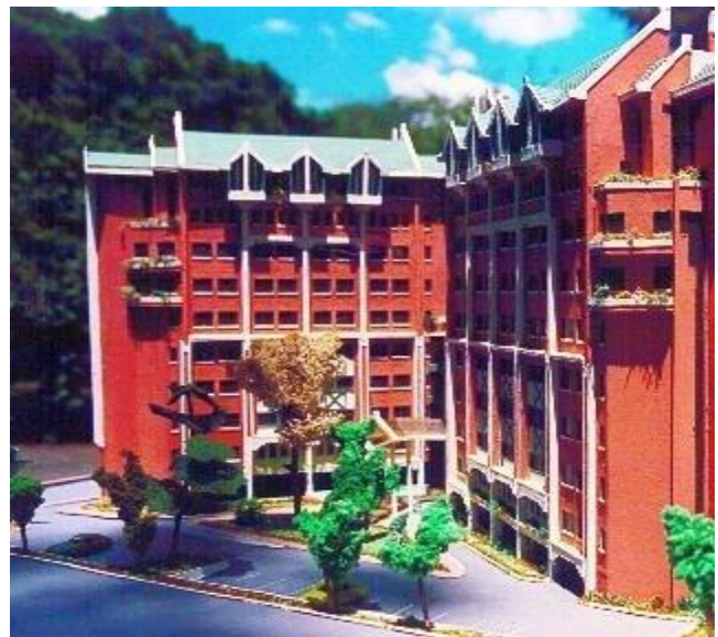
Fig. 22s. Architect unknown. The Chancery, Valley Road, Nairobi. s.a. The use of high roof pitches, cantilevers and 'warm' brick.
