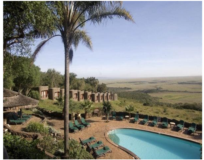
Fig 21h: Architect unknown, probably Symbion International. The Mara Sarova, Maasai Mara. s.a. A lodge that used the Manyatta as its referent in form genesis.
