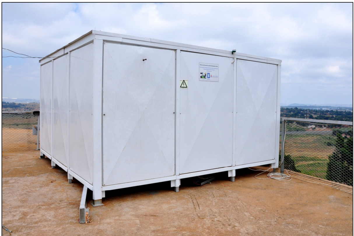
Figure 5-37: Pierre van Ryneveld turbine enclosure
