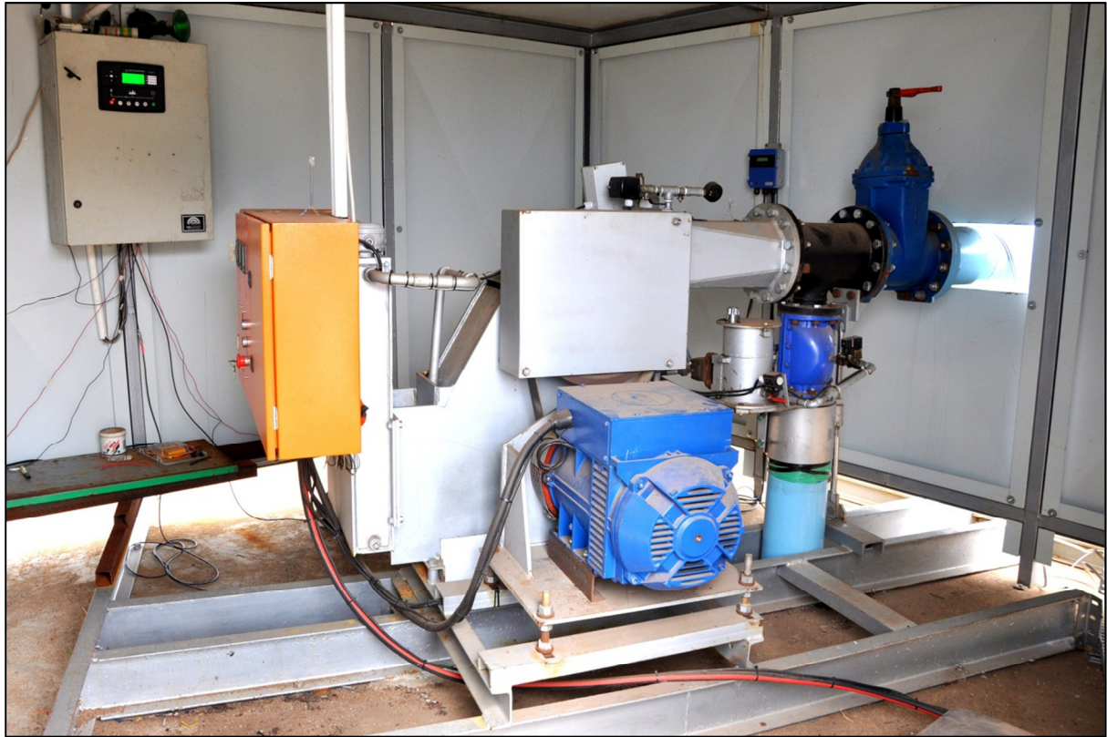
Figure 5-36: Completed turbine on steel-beam supports
