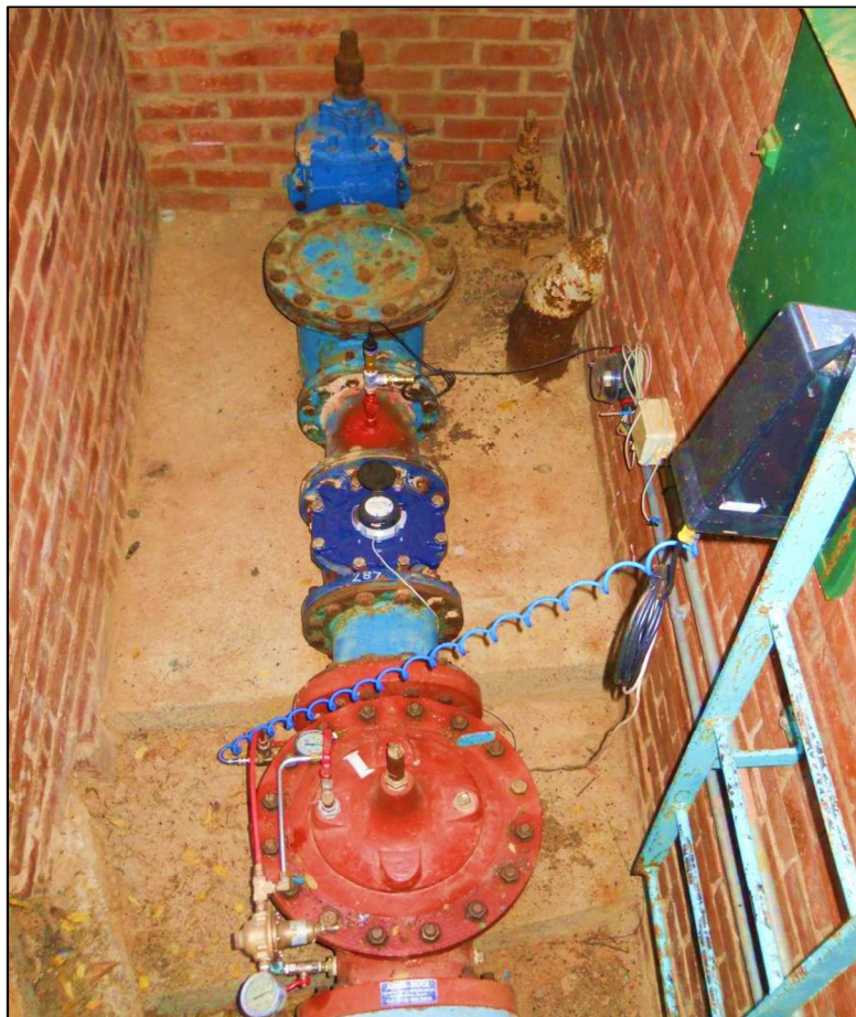
Figure 5-45: Pressure and flow measurement at Waterkloof pressure-reducing station
