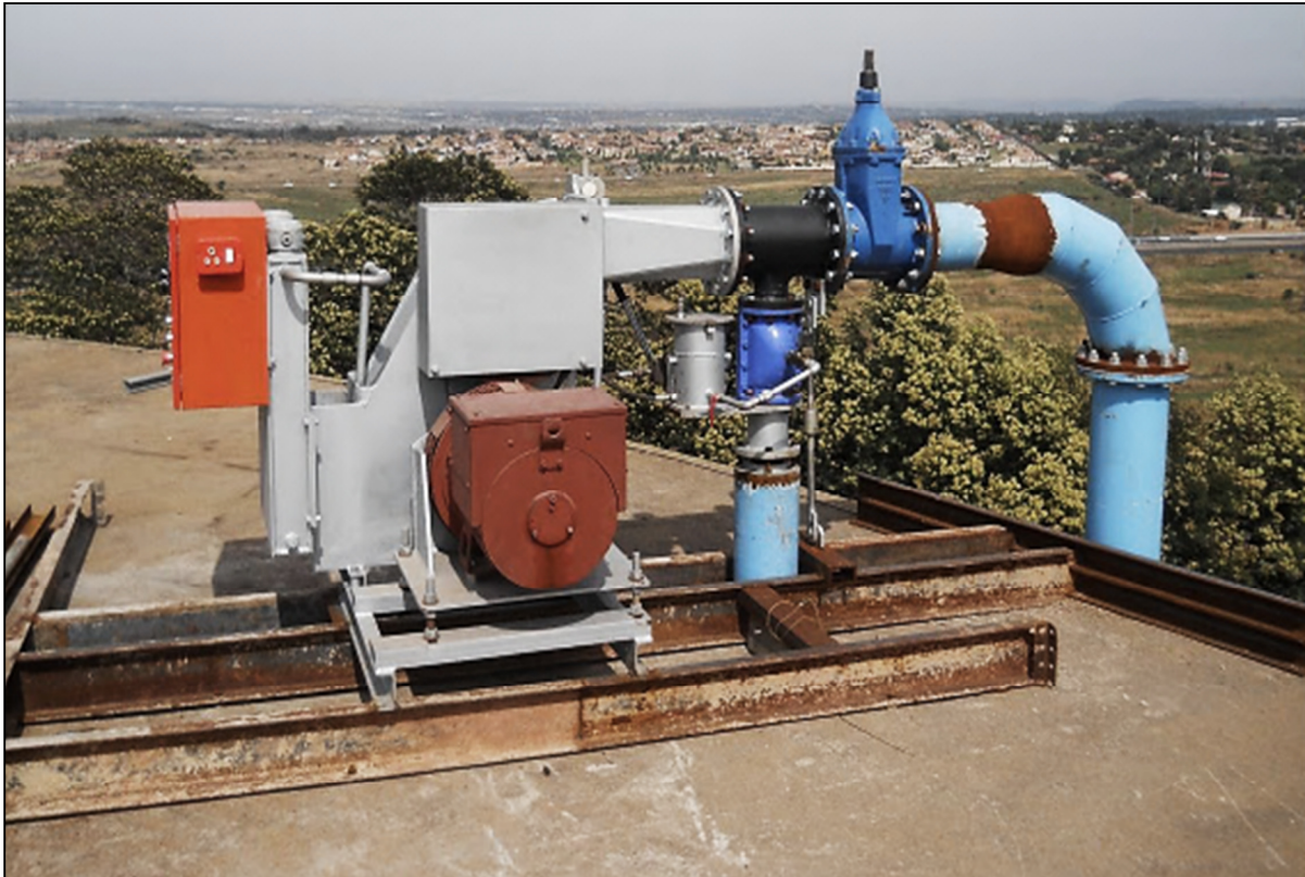
Figure 5-21: Existing Pierre van Ryneveld Reservoir hydropower installation
