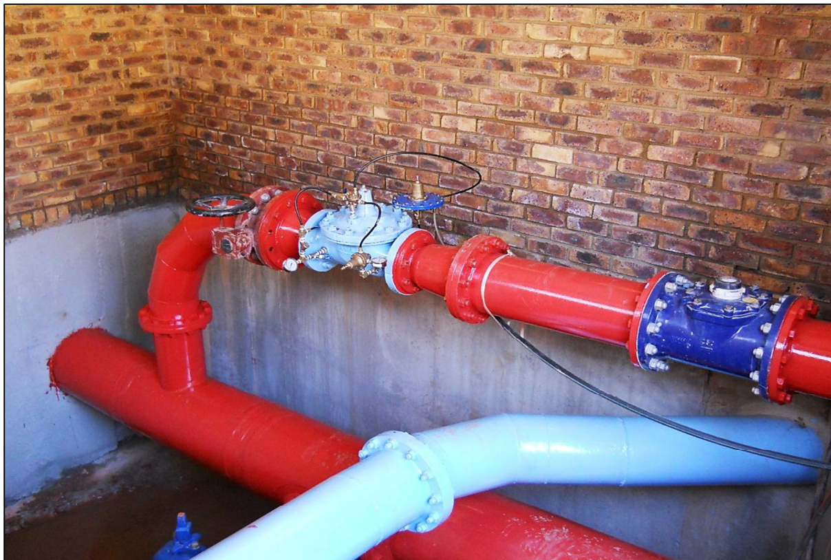
Figure 5-35: Completed off-take pipework
