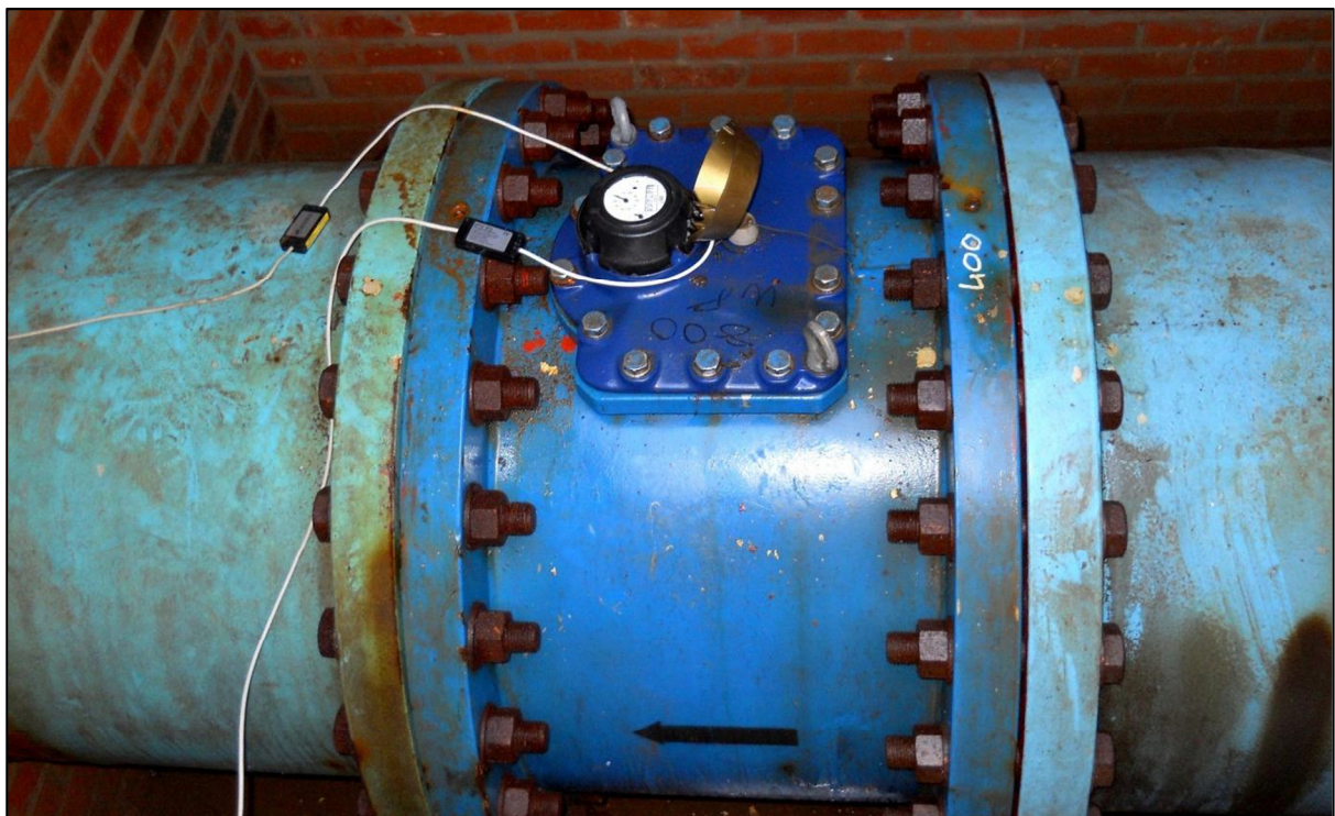
Figure 5-7: Flow measurement at Garsfontein Reservoir
