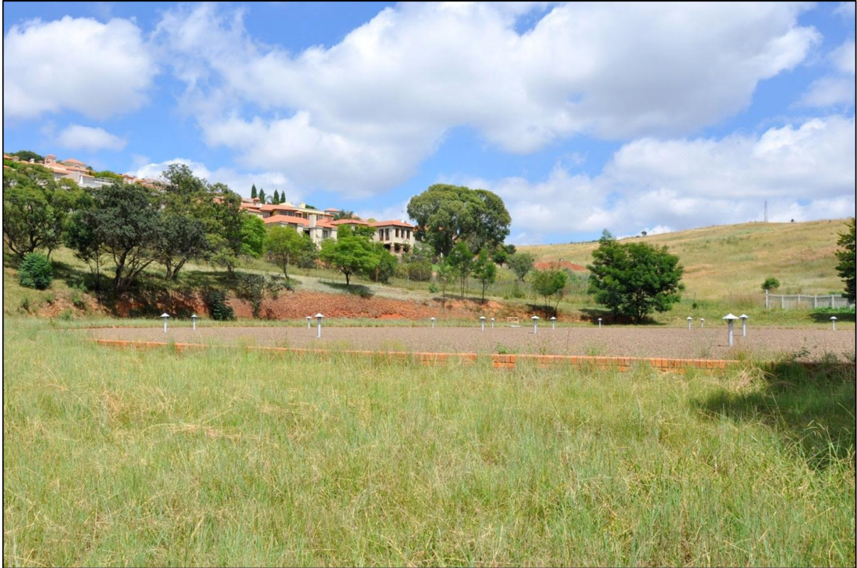
Figure 5-44: Waterkloof Reservoir roof
