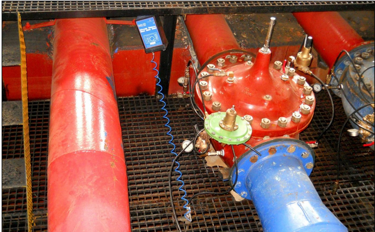
Figure 5-6: Pressure measurement at Garsfontein pressure-reducing station
