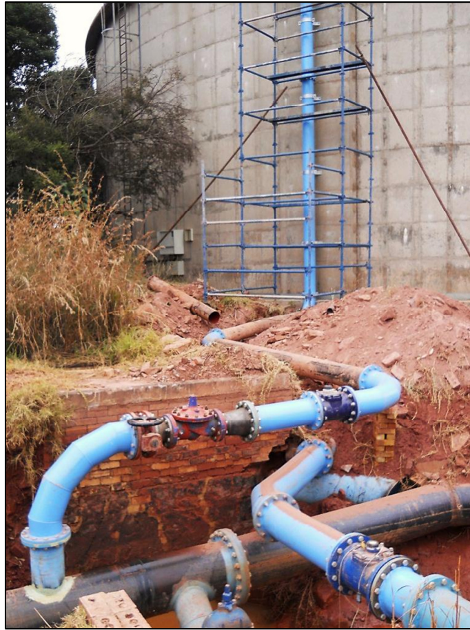
Figure 5-34: Pierre van Ryneveld off-take pipework under construction
