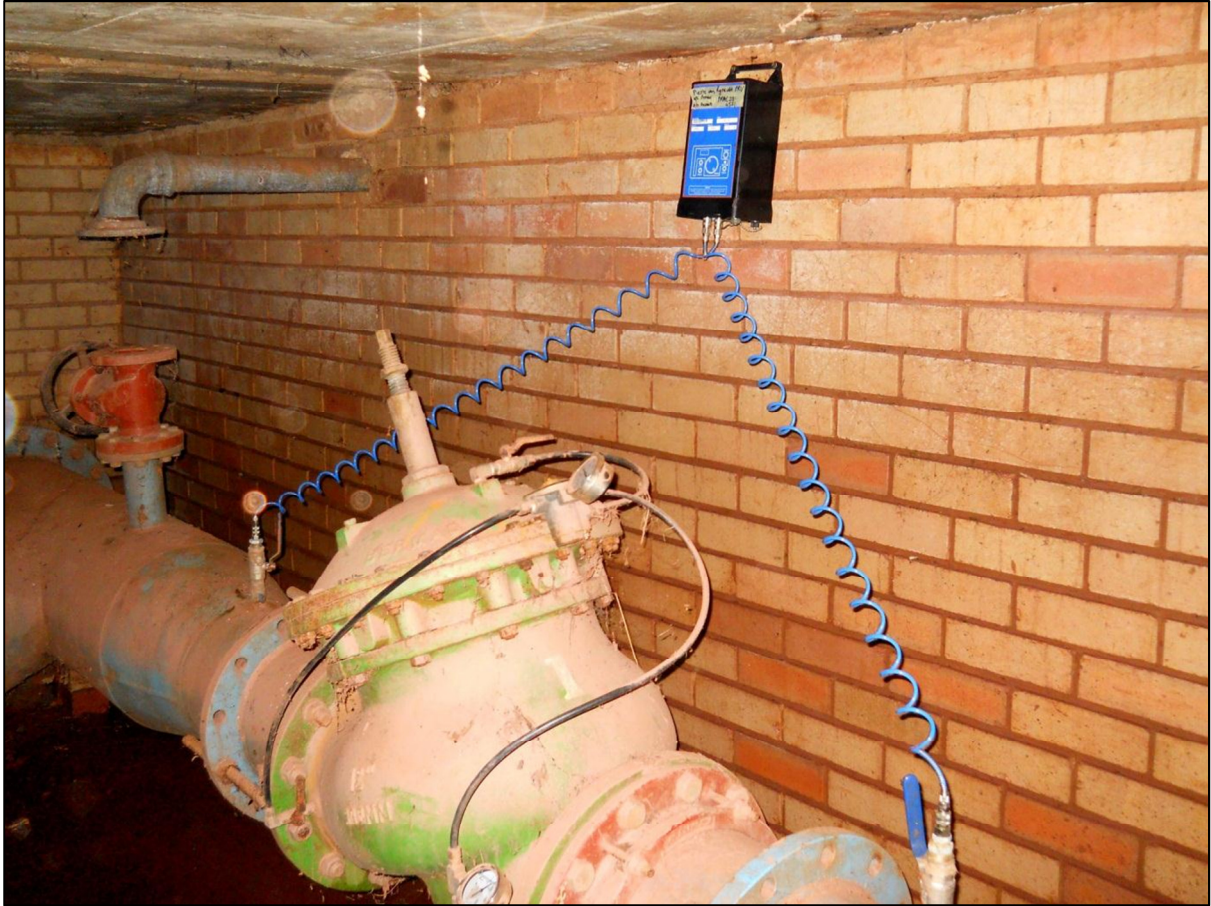
Figure 5-22: Pressure measurement at Pierre van Ryneveld pressure-reducing station
