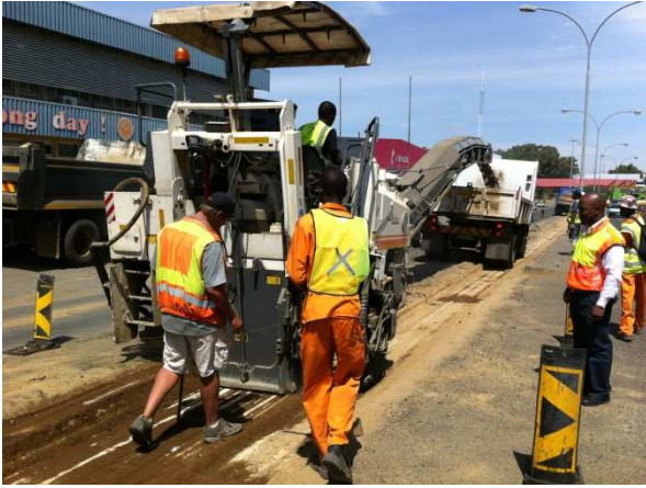
Figure 4: Milling out of existing base.
