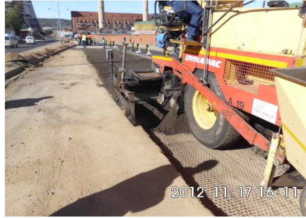
Figure 5: Paving of base.
