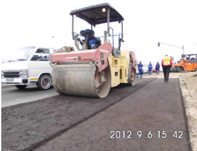
Figure 8: Rolling the base.
