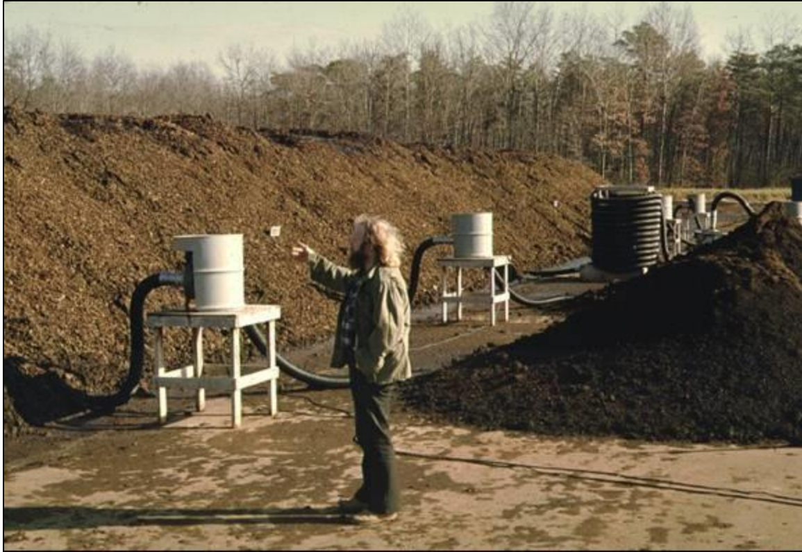
Figure 1.4 Sewage sludge and wood chip feedstock being composted by a static (unturned), aerated pile/windrow method. Air is drawn through the windrow via perforated pipes connected to small blowers and expelled through piles of finished compost that absorb odours (Brady and Weil, 1999)
