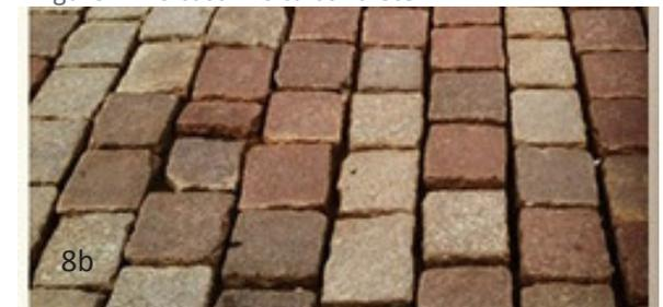
Figure. 7.11 Cobblestone paving
