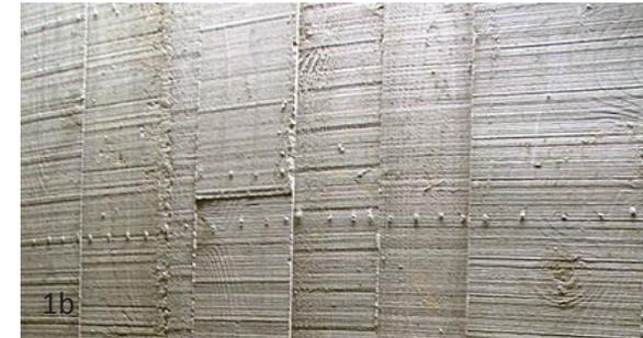
Figure. 7.2 Timber off-shutter finish
