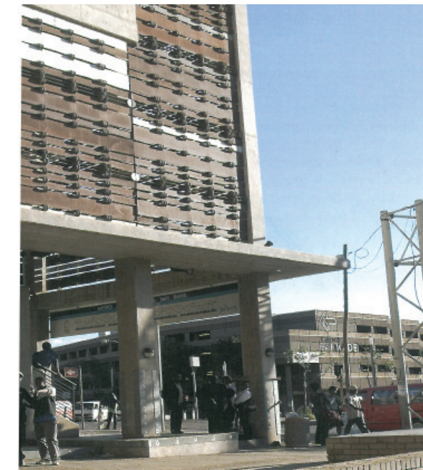
Image 6.11. Metro mall entrance structure
