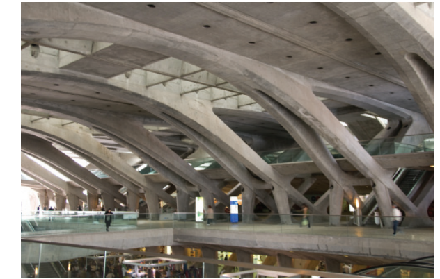
Image 6.16. Oriente Station ground floor concrete structure
