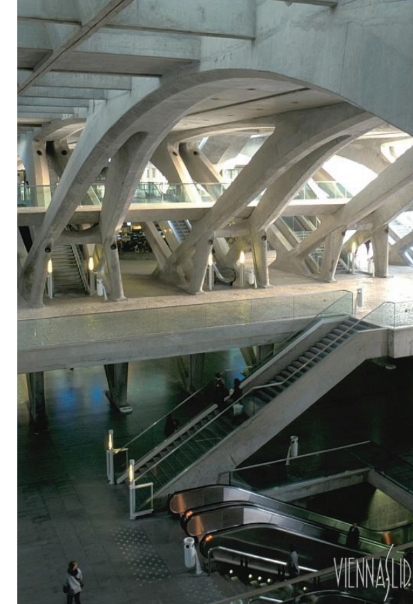
Image 6.14. Oriente Station main transfer space
