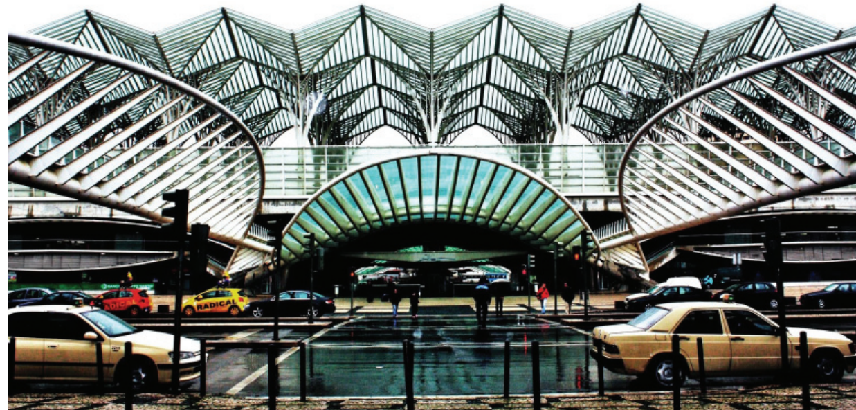
Image 6.13. Oriente Station main entrance
