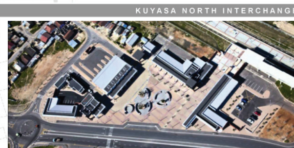
Image 6.5. Kuyasa Station aerial view
