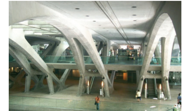
Image 6.17. Oriente Station Double volume entrance area
