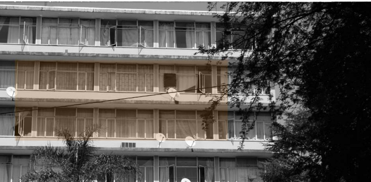
Figure 72: Apartment block across the street at Lillian Ngoyi Street (Author 2013)
