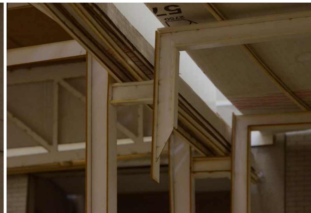
Figure 299: Model 2: suspended portal frame details: portals between activity zone and spectator zone (Author November 2013)
