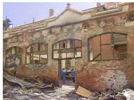
Figure 118: Damage caused by fire (Unknown)
