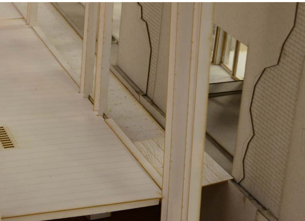
Figure 297: Model 2: floor details: new multi-sports hall, connecting charred timber walkway, separation articulated with recessed concrete tiles and existing western passage floors (Author November 2013)
