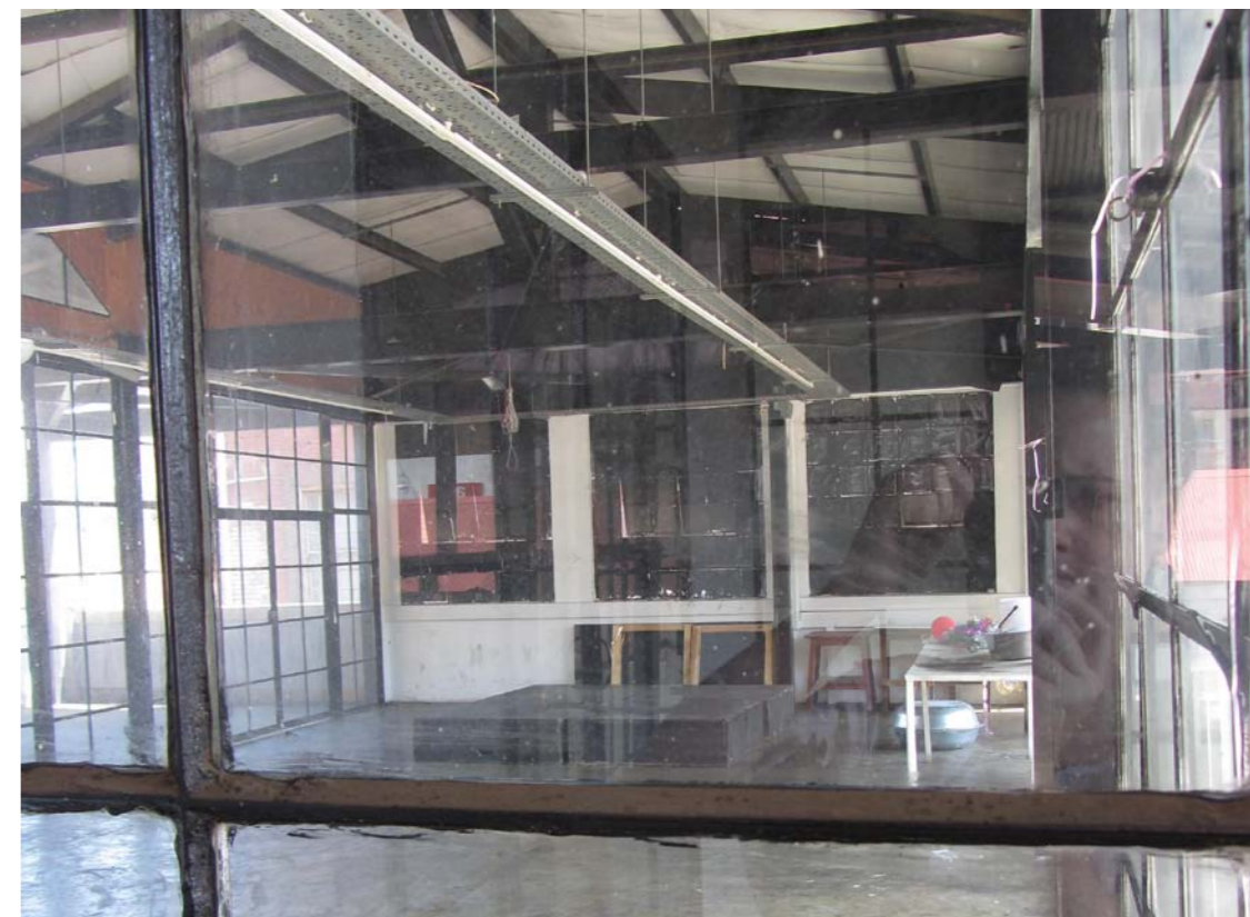
Figure 120: Vacant interior (Wilkinson 2012)
