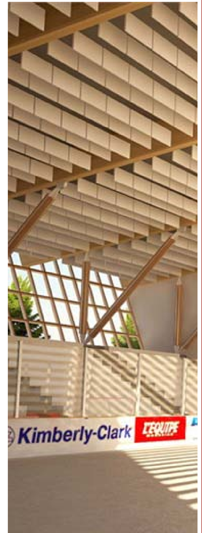
Figure 215: Acoustic baffles (Rockfon 2012)
