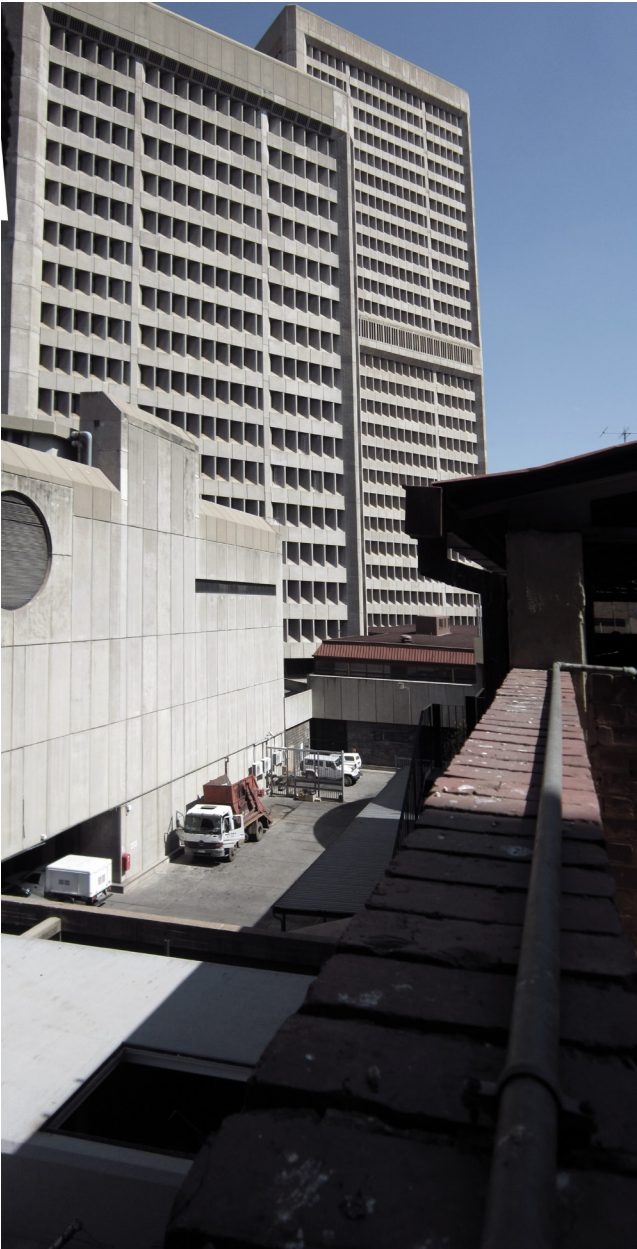
Figure 21: Service yard behind Telkom Call Centre (Author 2013).
