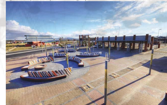
Fig 05-16 Kuyasa Transport Interchange space defined by the building
