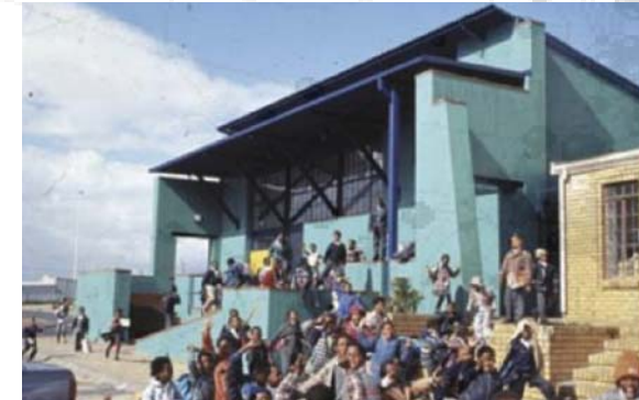
Fig 05-2 Khayelitsha Service Centre and Pay Point is a centre for the community
