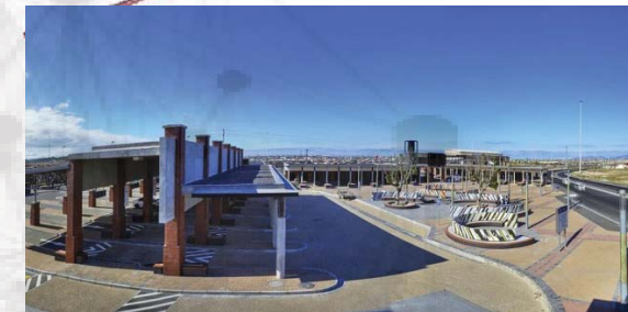
Fig 05-14 Kuyasa Transport Interchange taxi rank structures
