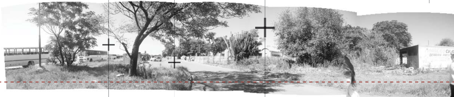
Panorama view of the taxi rank and station from the west
