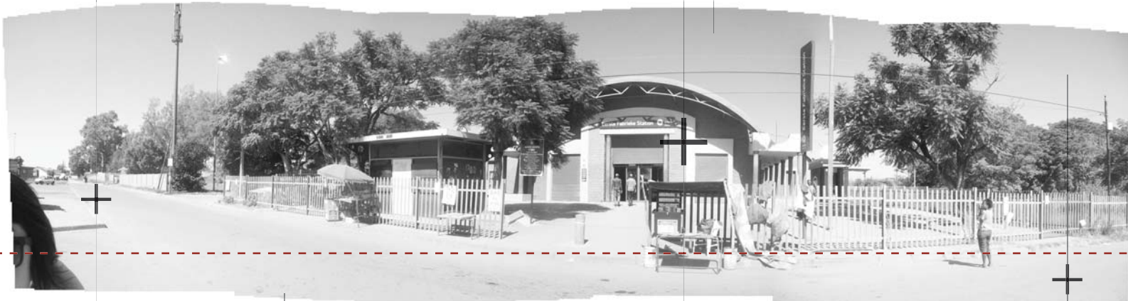
Panorama view of Station from the north
