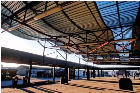
Fig 05-7 Central Meat Market truss structure
