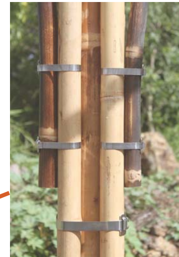
Fig. 108: Bamboo Column Detail
