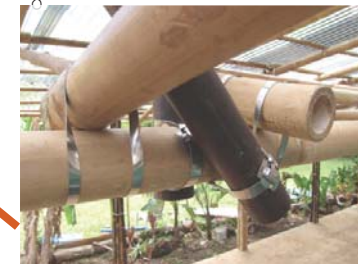
Fig. 110: Bamboo truss connection detail
