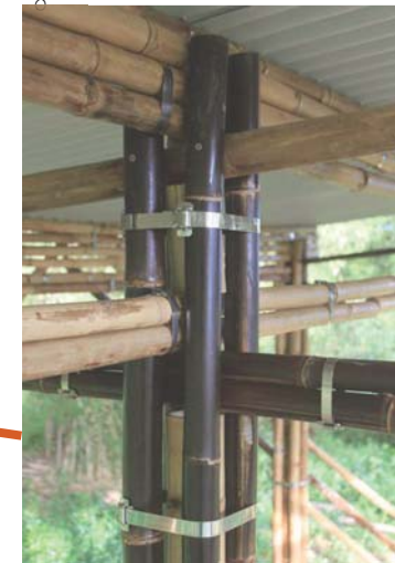
Fig. 109: Bamboo column/truss detail
