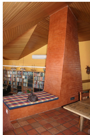
8. Detail of chimney
