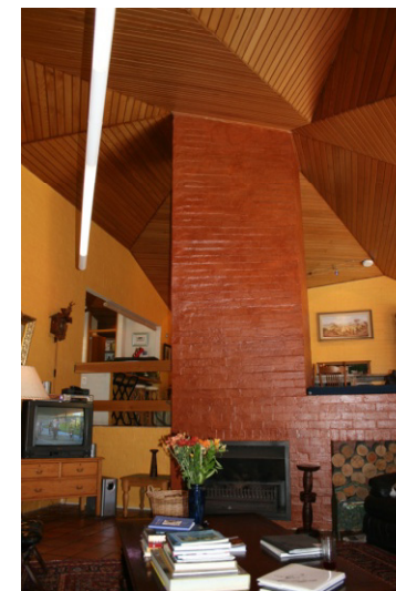
9. View of chimney below roof
