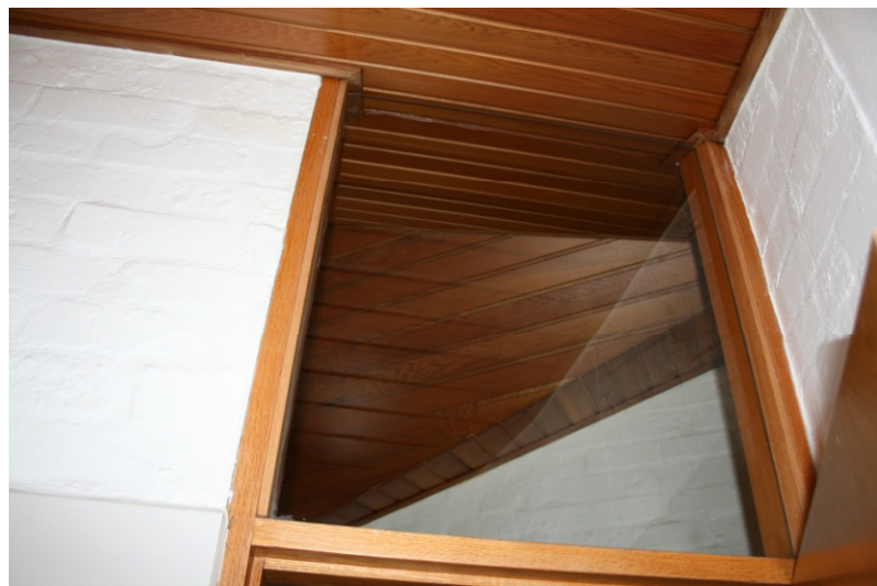
7. Detail of door head below roof
