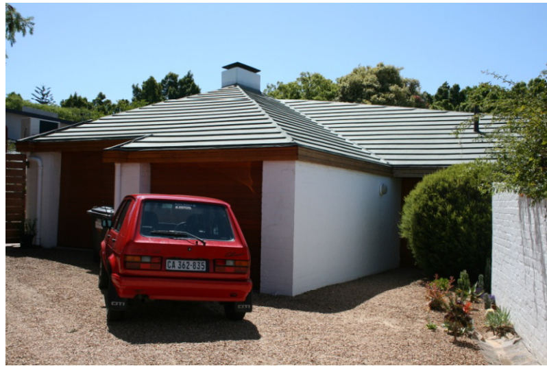
1. View from the driveway looking west
