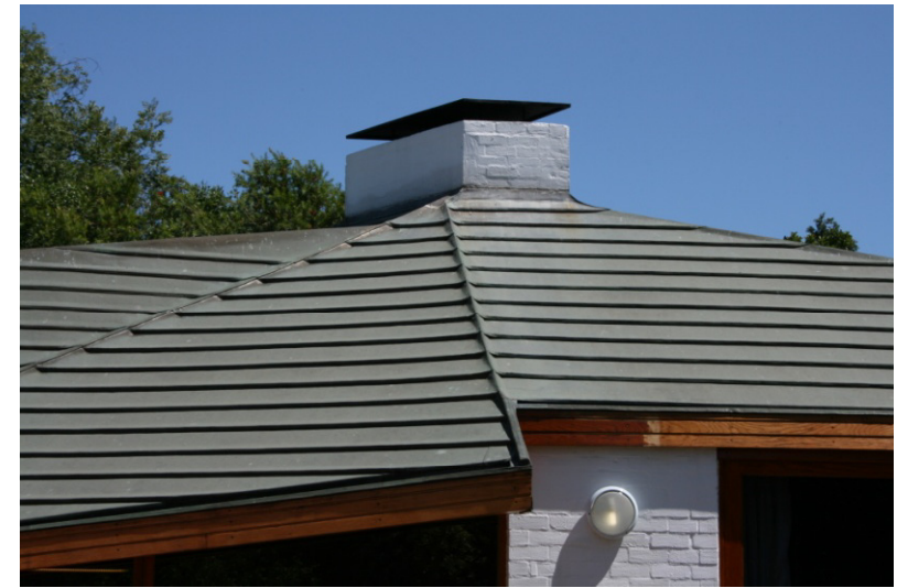
3. View of the roof from the garden
