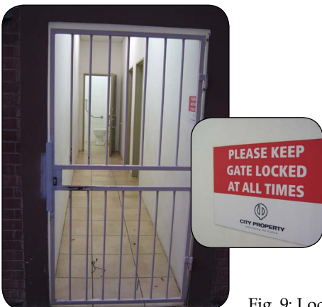
Fig. 9: Locked public toilets
