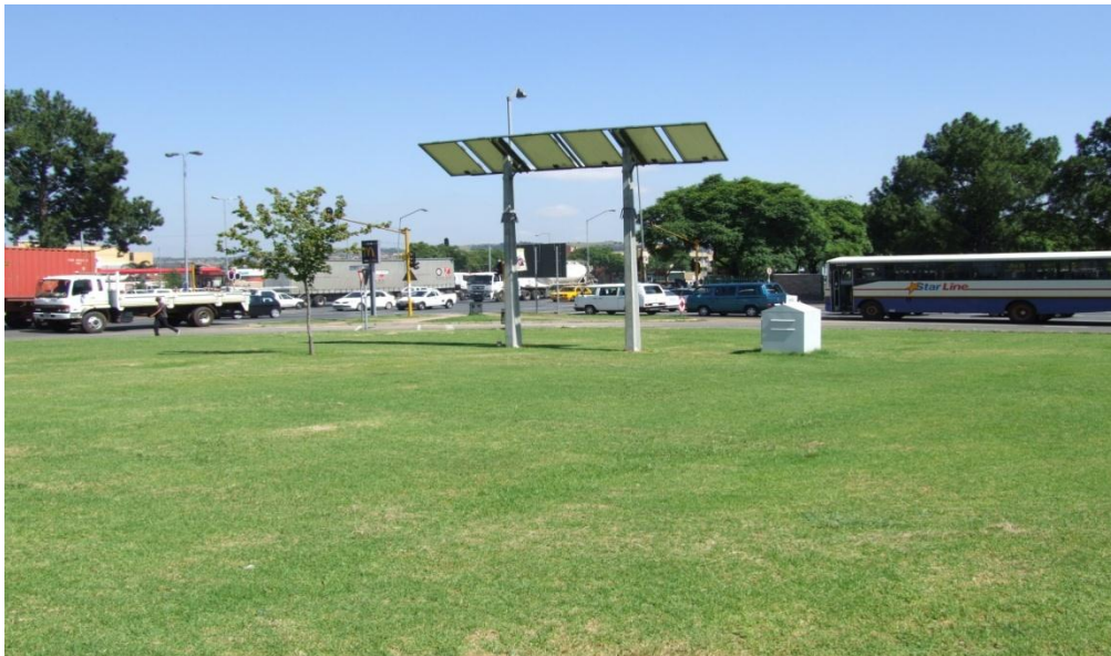
Figure 3.5: Traffic light on corner of DF Malan and Church Street operating by solar energy
