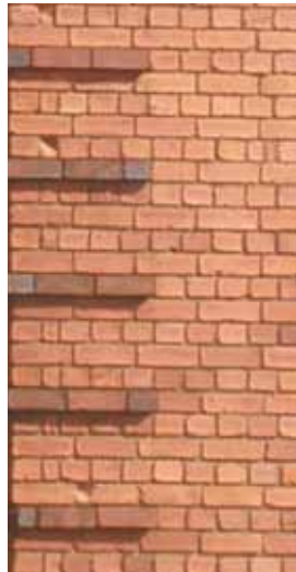
PLASTERED DIVISION BETWEEN MASONRY AND WALL AND ROOF
