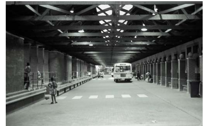
Fig.5.12: Interior view of host building with bus passing through (Marnus Barnard).
