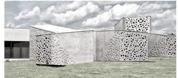
Fig.6.55: Day view of exterior (Lerouge, 2010)
