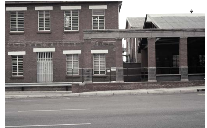
Fig.5.6: Exterior view of bus entrance into host building. Note that the steel columns have been clad with brick layers (Marnus Barnard, 1993).
