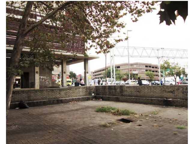
Fig.6.25: Empty exterior courtyard (Author:2012)
