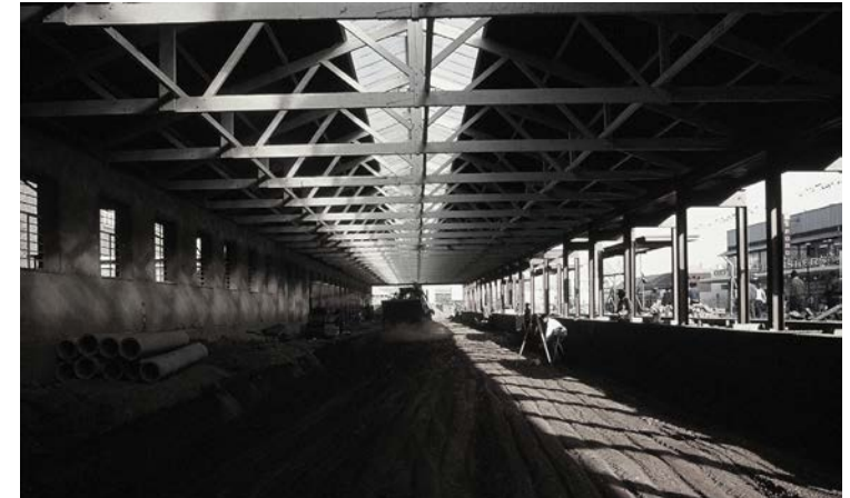
Fig.5.9: Interior view of construction process. Excavation of interior floor (Marnus Barnard).
