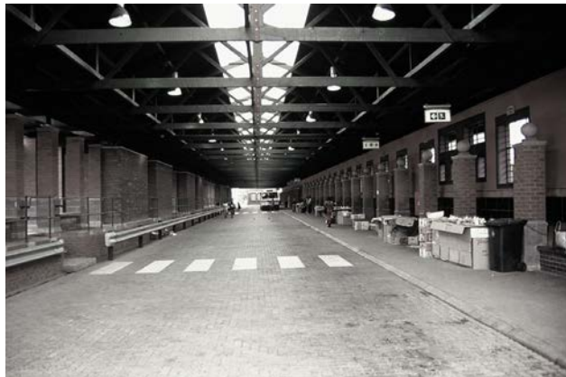
Fig.5.11: Interior view of host building (Marnus Barnard).
