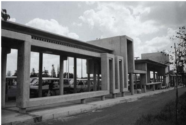
Fig.6.4: Seating niches provided in concrete arcade (Deckler et al. 2006).
