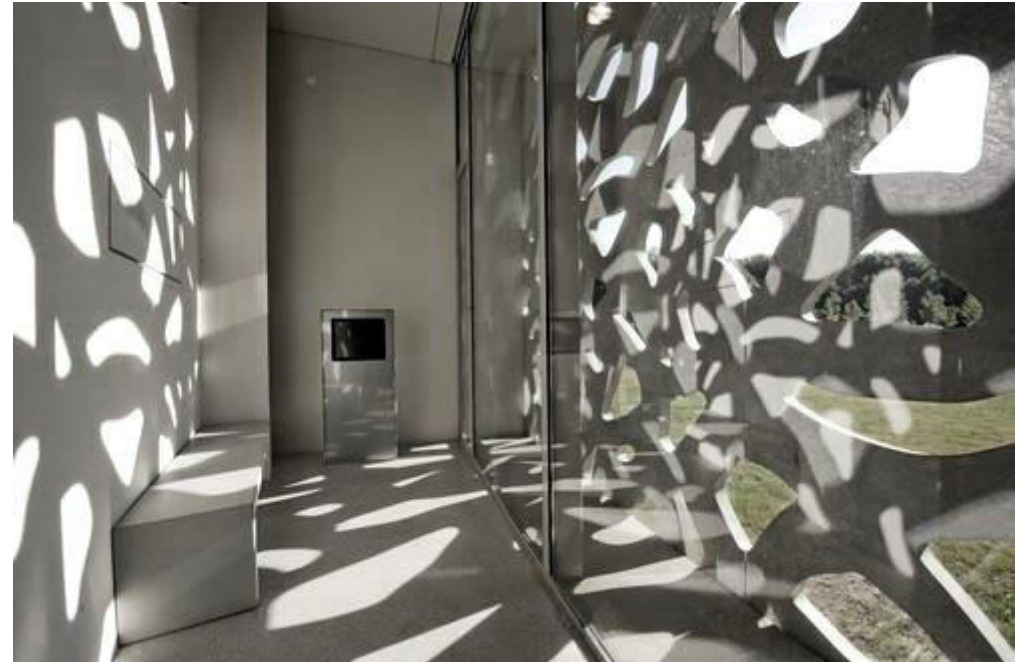
Fig.6.57: Interior view of perforated concrete screen (Lerouge, 2010)
