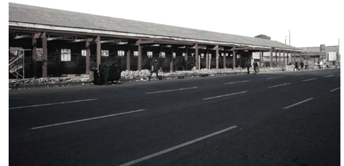
Fig.5.5: Alteration of northern facade (Marnus Barbard, 1993).
