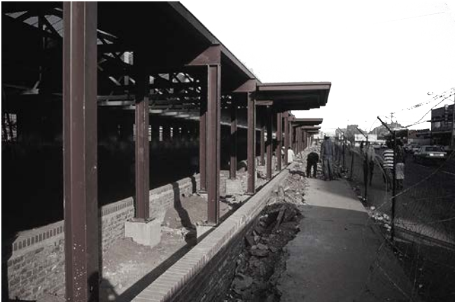
Fig.5.8: Northern edge alteration with steel columns for shops (Marnus Barnard, 1993).
