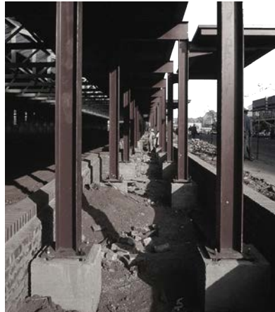
Fig.5.7: Steel columns where shops are to be situated (Marnus Barnard).
