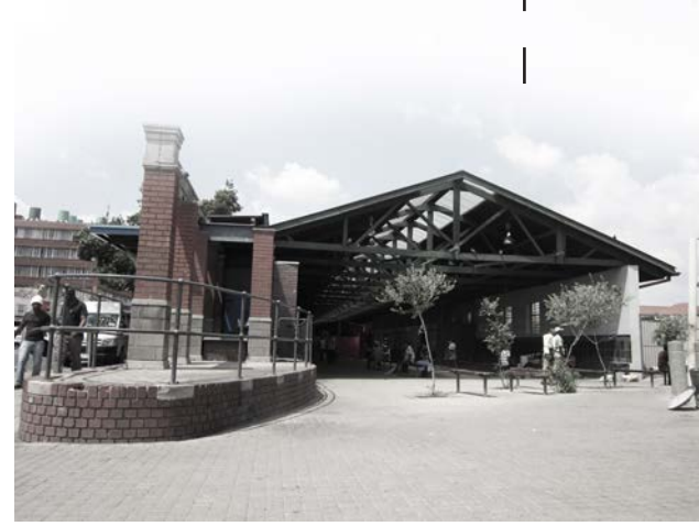
Fig.8.8: Existing western entrance (Author, 2013).
